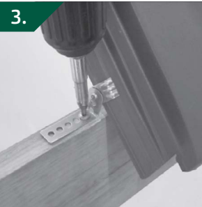
3. Place twisted tip of the clip onto the sidelock and screw it into the fascia board.
