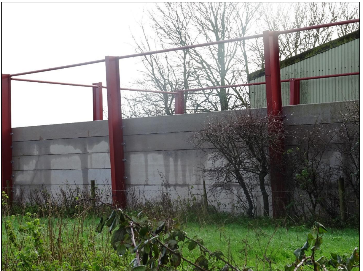
Close up view, from North Farmhouse boundary.
