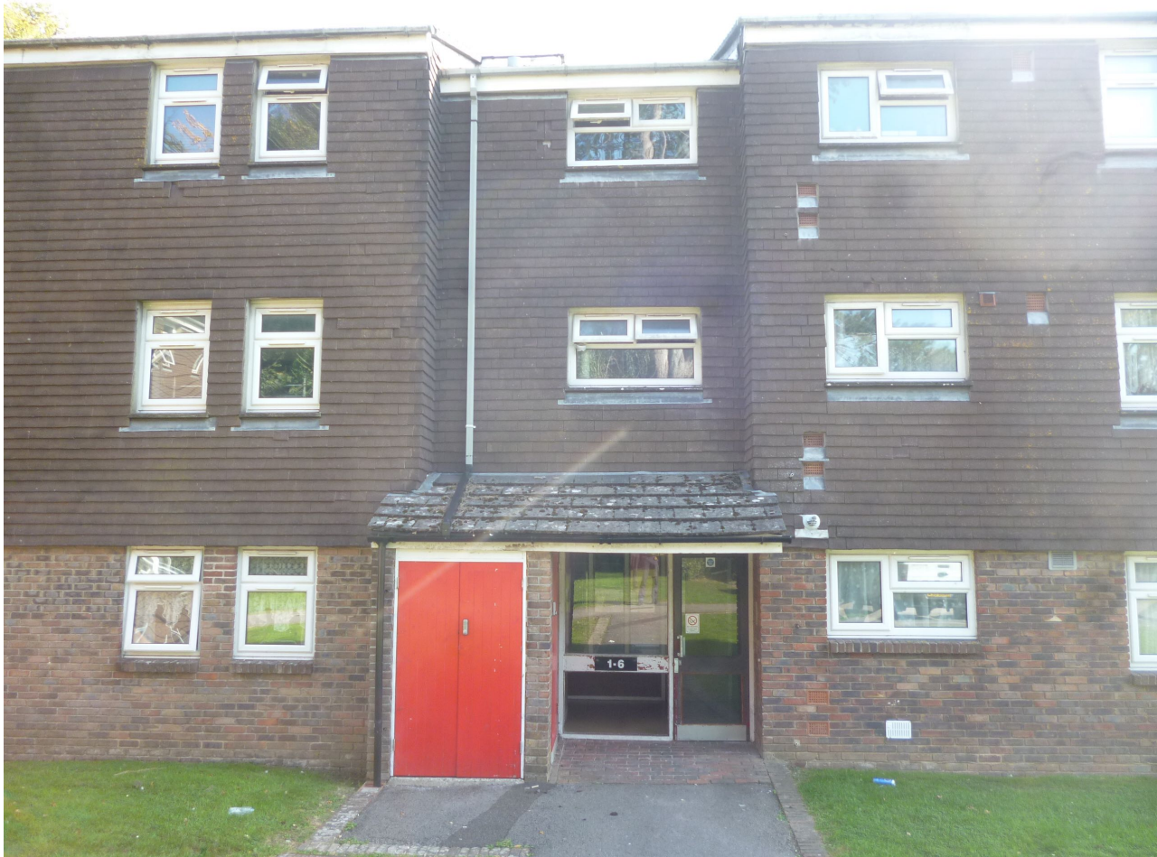
Existing Front Elevation Image
