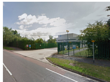
No.1 - View looking north east to the existing most southern access junction.
