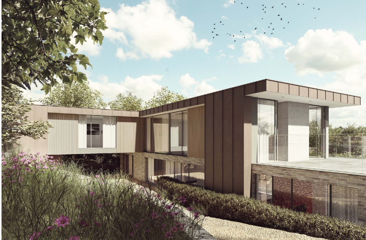
Quarry Road (Re-Format LLP)
