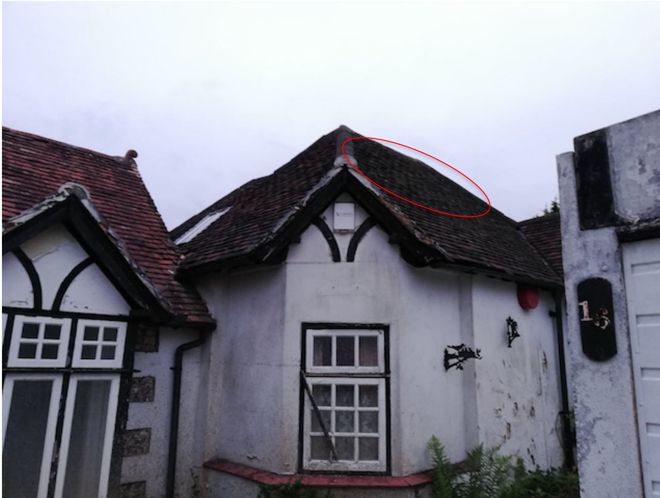
Figure 4. Approximate location of the Common Pipistrelle emergence during the first survey
