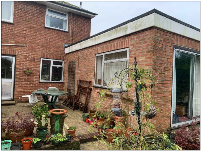
REAR SHOWING EXISTING CLIENT EXTENSION
