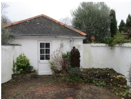
Fig 10 – Garage façade facing into the rear courtyard
