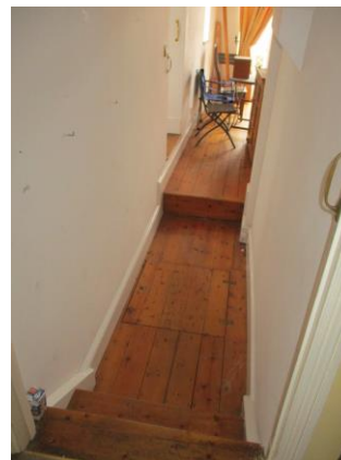
Fig 4 -View of the existing stepped access under the stairs to the rear of the property with existing cellar hatch visible.
