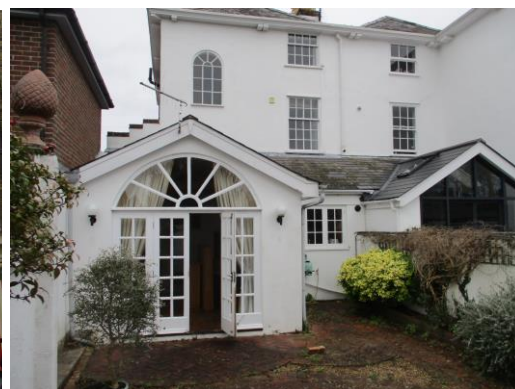
Fig 2 - Rear elevation, viewed from rear terrace
