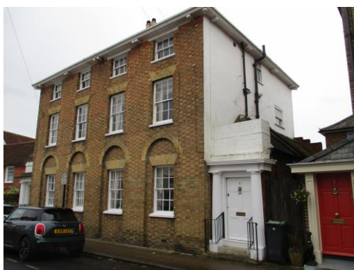
Fig 1 – Front elevation, viewed from King Street
