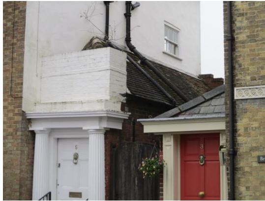
Fig 9 -View of the existing pitched roof above the hallway
