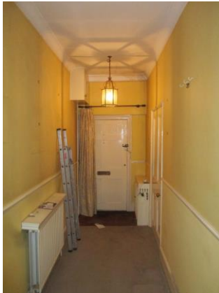
Fig 8 – View of the existing hallway.
