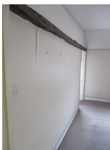
Fig 6 - View of the existing ceiling tie/partition wall in Bed 2
