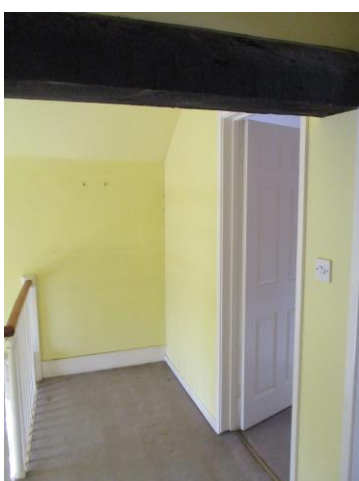
Fig 5 – View of existing second floor landing
