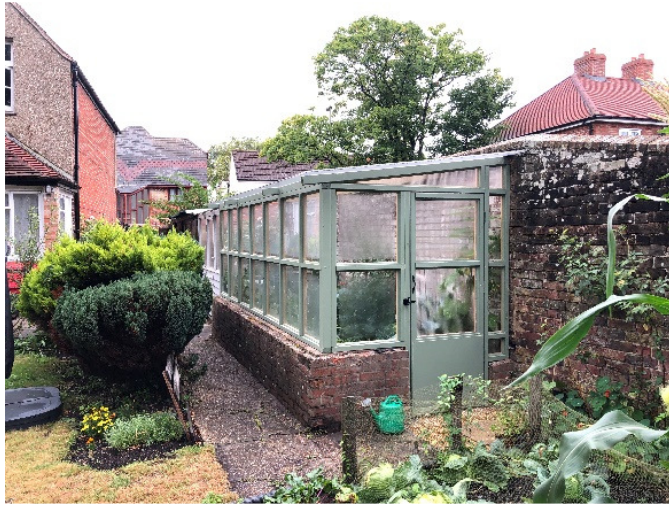
Figure 1, existing outbuildings to be retained.
