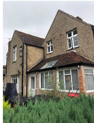
Figure 2, existing conservatory to be demolished and re-built in new proposal.
