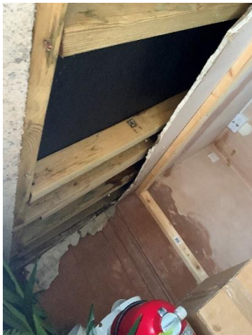
Photo of the internal structure of the existing store
