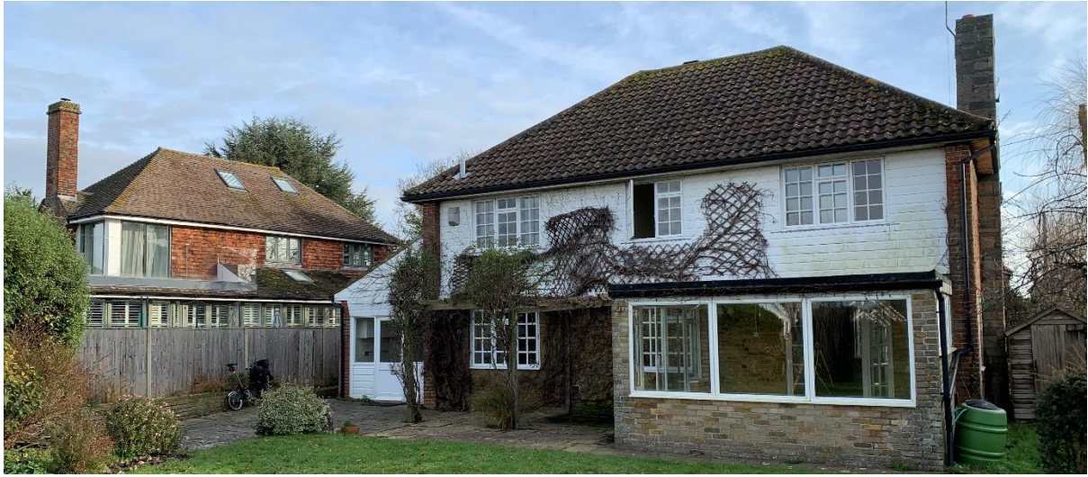
Rear of Dwelling – plastic cladding being removed. Rear single storey extension across the back – the mono pitched roof to the left of the photo will extend out to improve privacy to the immediate rear of the dwelling
