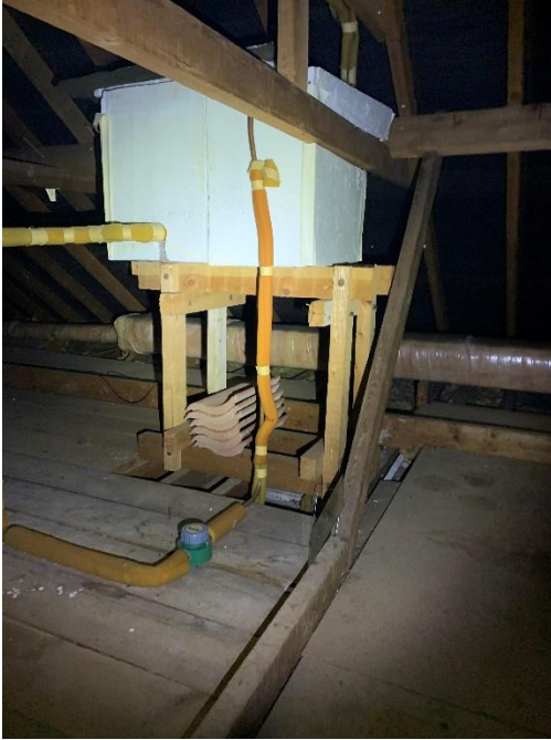
Attic and tanks
