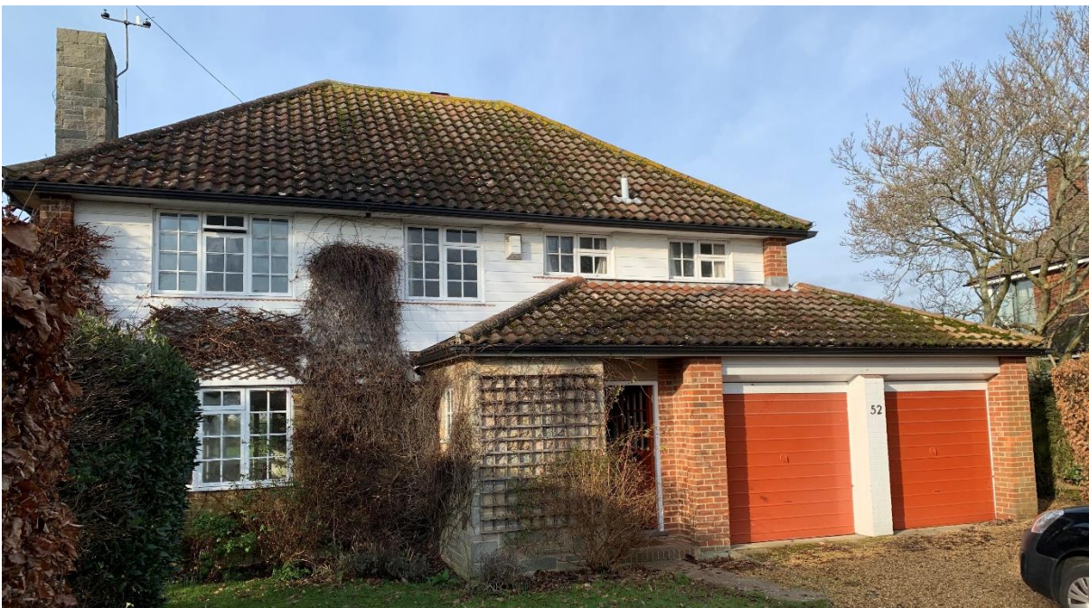
Front of dwelling – white plastic cladding being replaced with timber. Orange/ brown garage doors will become 2 smaller windows and walls to be insulated and have through colour render applied.
