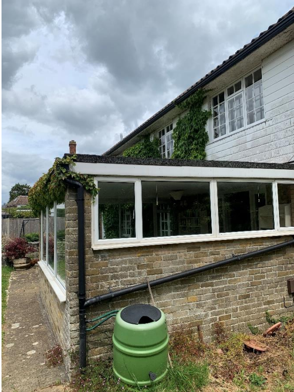
Rear Flat roof extension being removed. Note white plastic cladding above also being replaced with timber.
