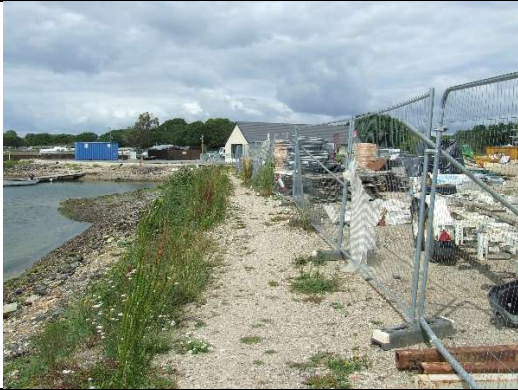
Looking west towards the site – area of sea wall to be cleaned up in the foreground, slipway to the middle.
