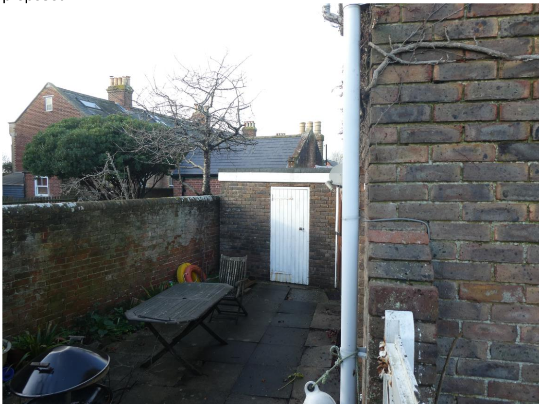
Rear south elevation of garage to be demolished, photograph from within curtilage.
