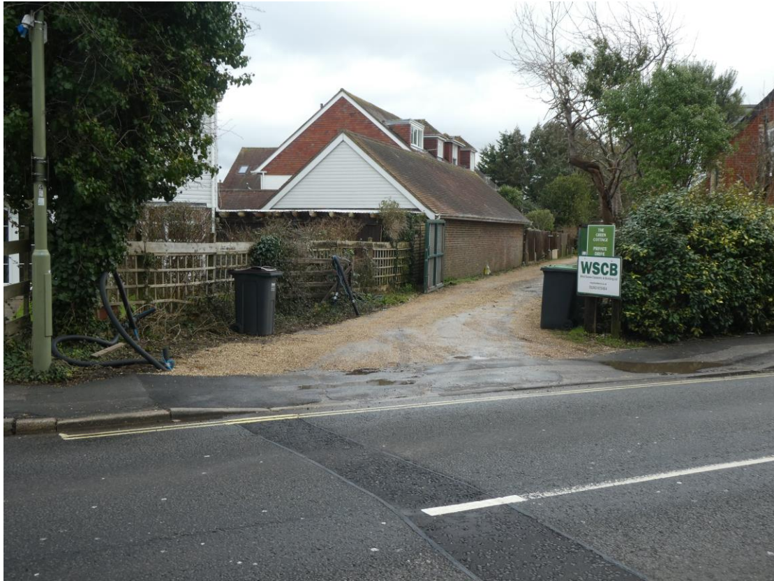
Access to Langstone Road. Building Contractors temporary security gates.
