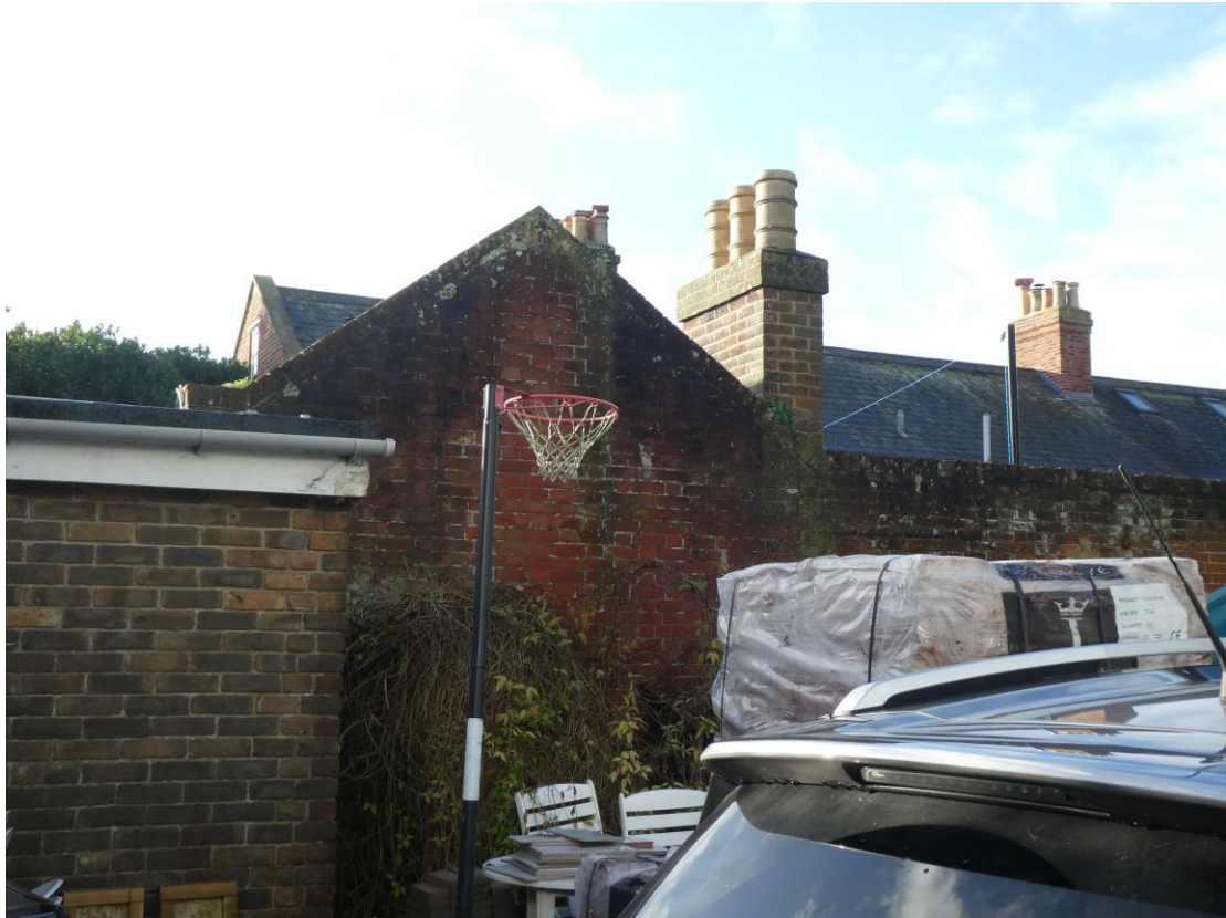
Left part flat roofed garage to be demolished, high boundary wall and adjacent outbuilding.
