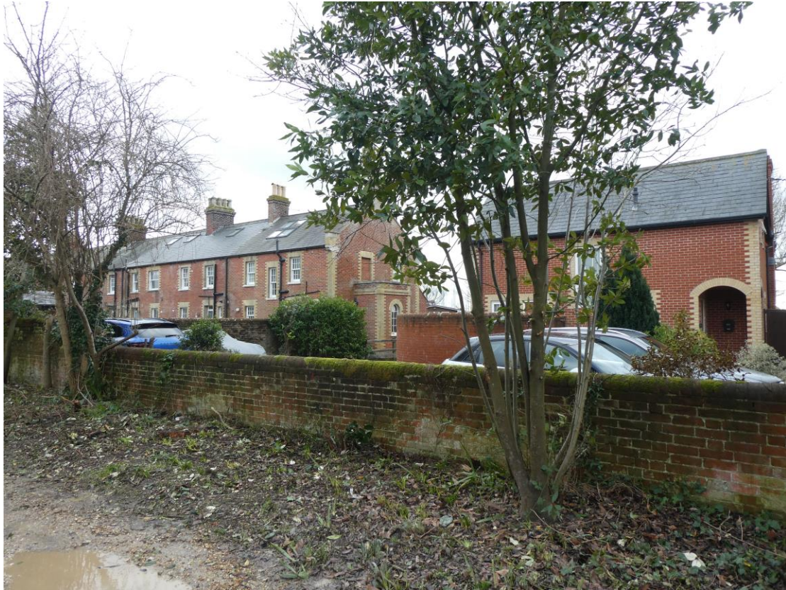
Boundary wall to the rear of 77 Langstone Road and communal area with parking spaces.
