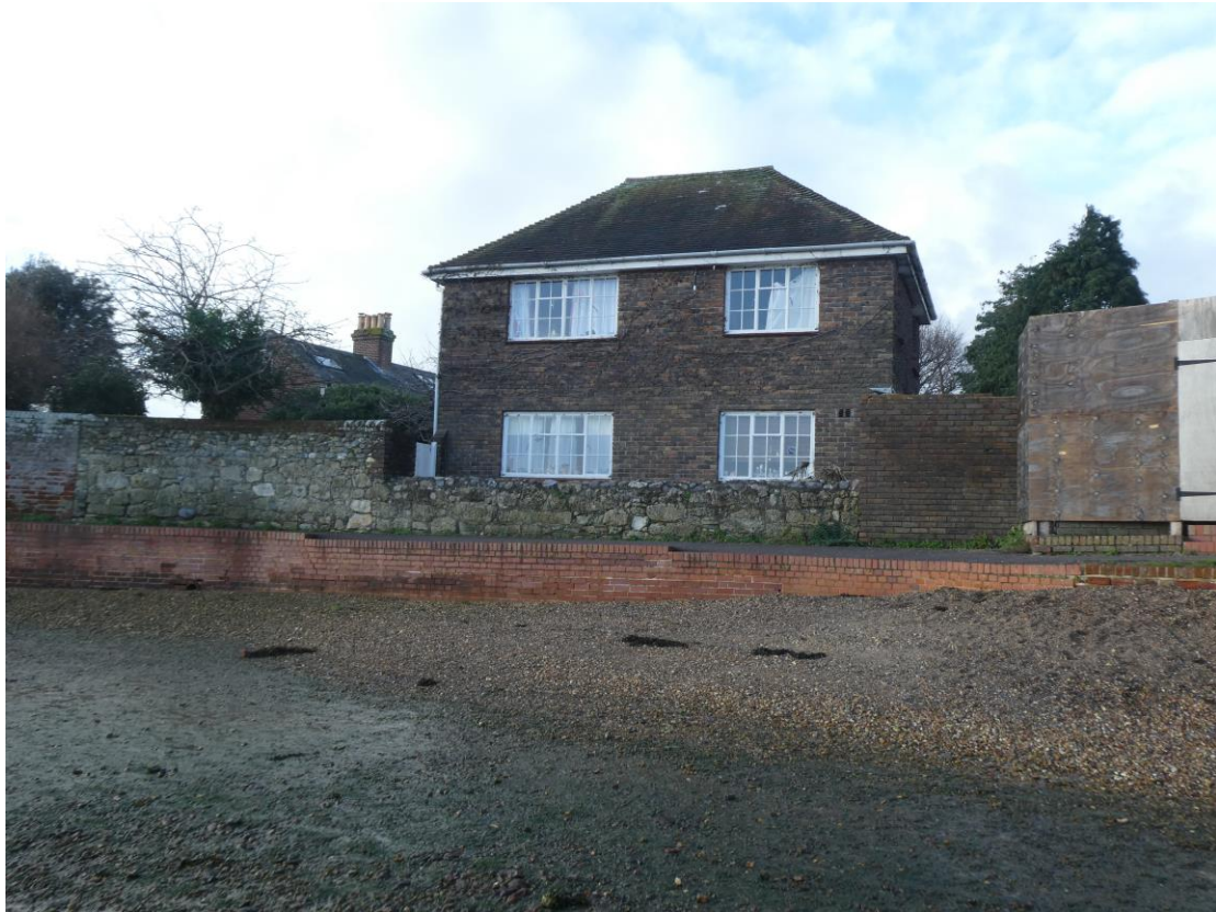
Annexe east elevation steel windows.
