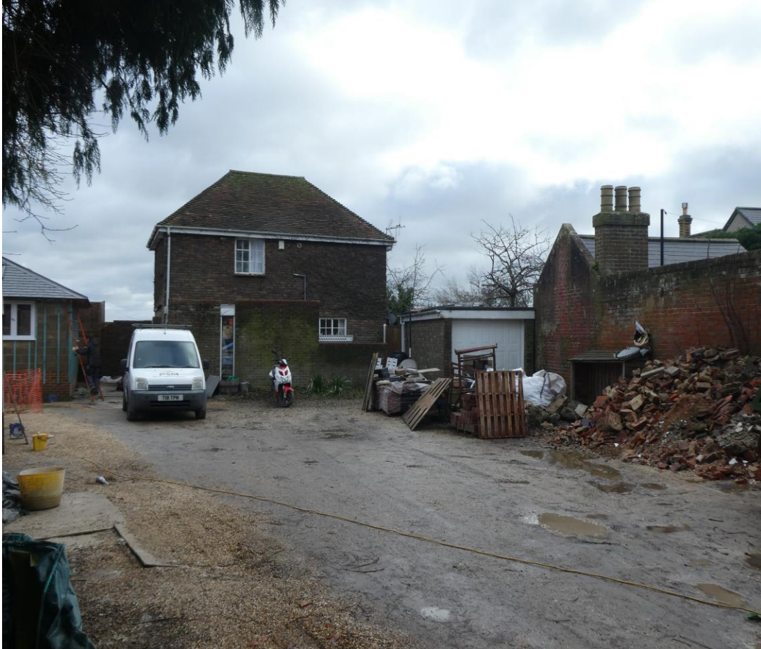
Rear (west) elevation of the annexe, garage to the right to be demolished.
