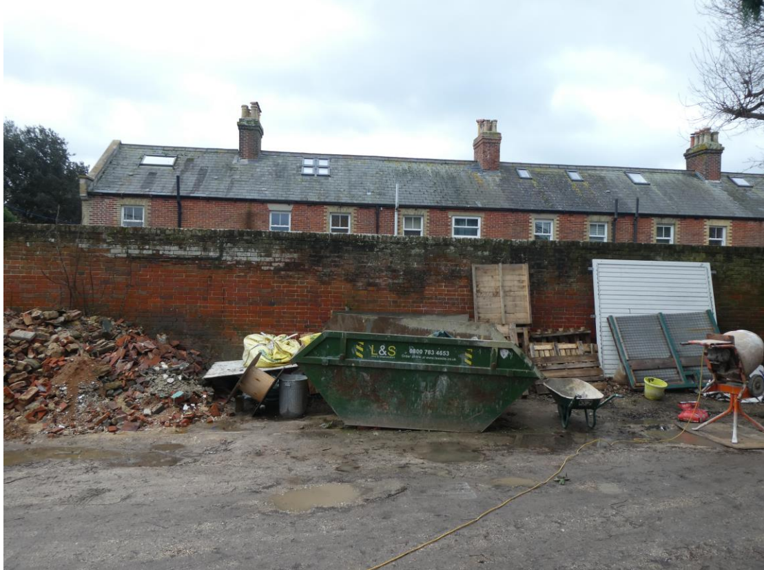
Boundary wall to the rear of Coastguard Cottages, temporary builders work.
