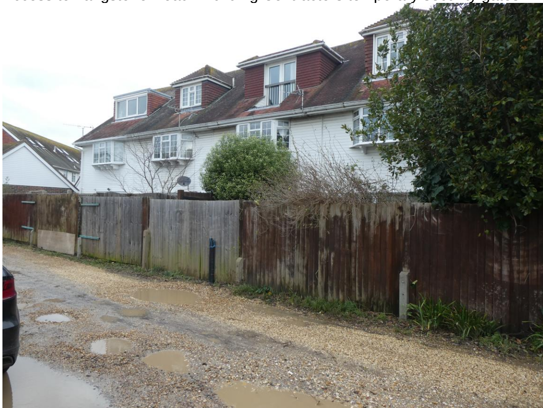
North side of vehicular access drive, rear of Tower Garden dwellings.
