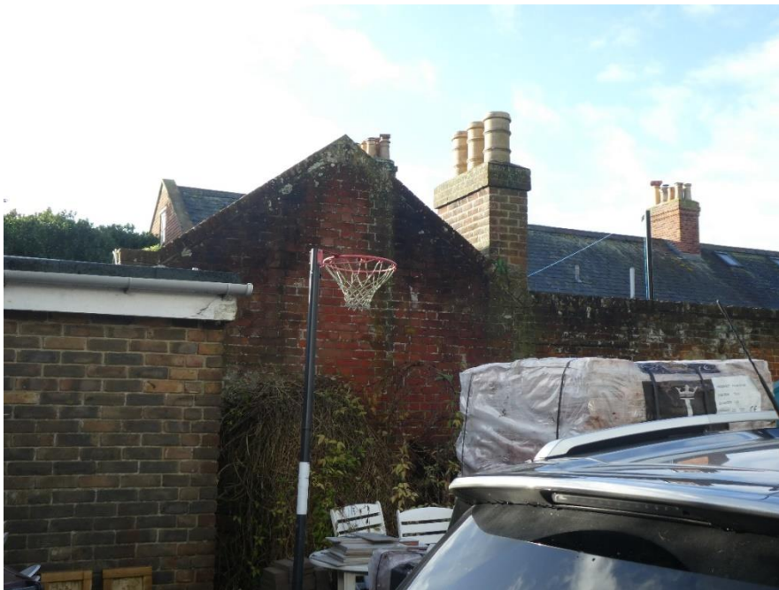
BOUNDARY WALL BETWEEN THE GREEN COTTAGE & COASTGUARD COTTAGES, ADJACENT OUTBUILDING WITH CHIMNEY.
