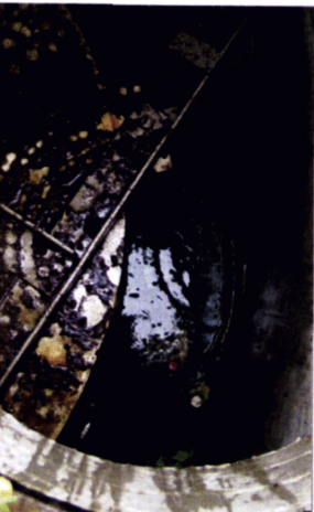
Fig 8 View of outer annulus of floatables and oil collection zone.
