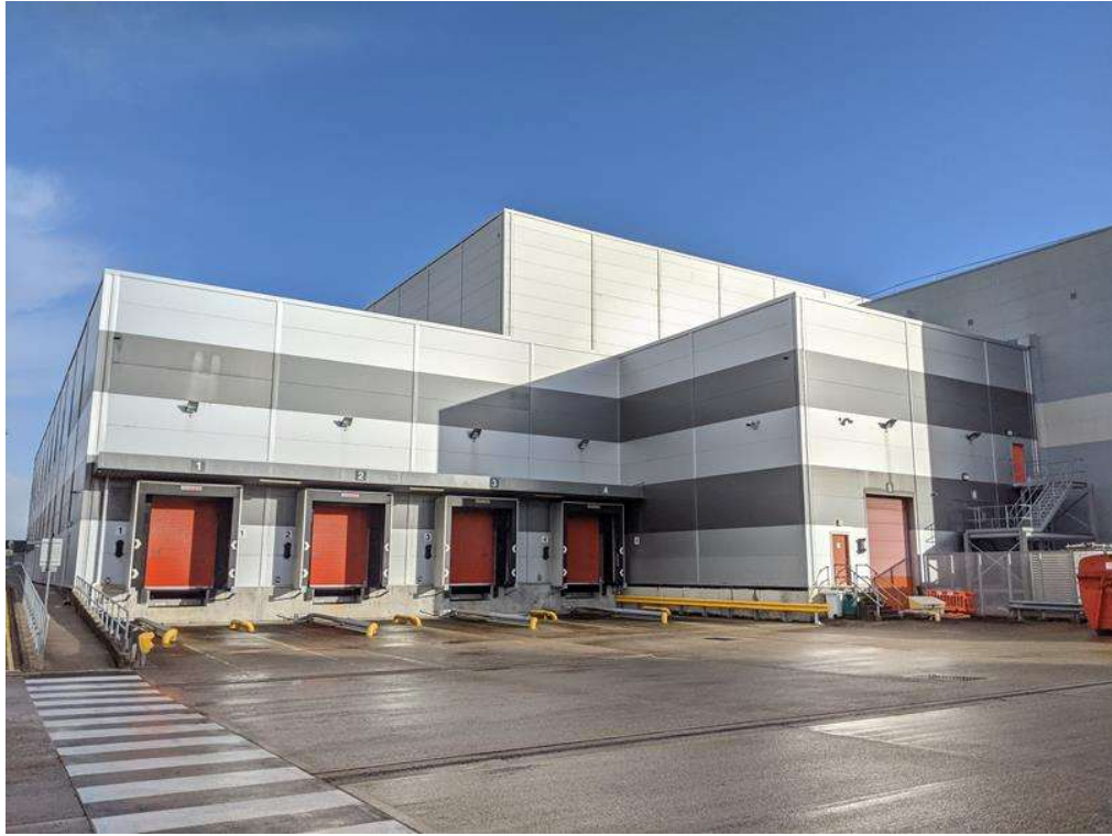
Photo 1 – Buildings on-site offer negligible bat roost potential but should be checked for nesting gulls prior to demolition.
