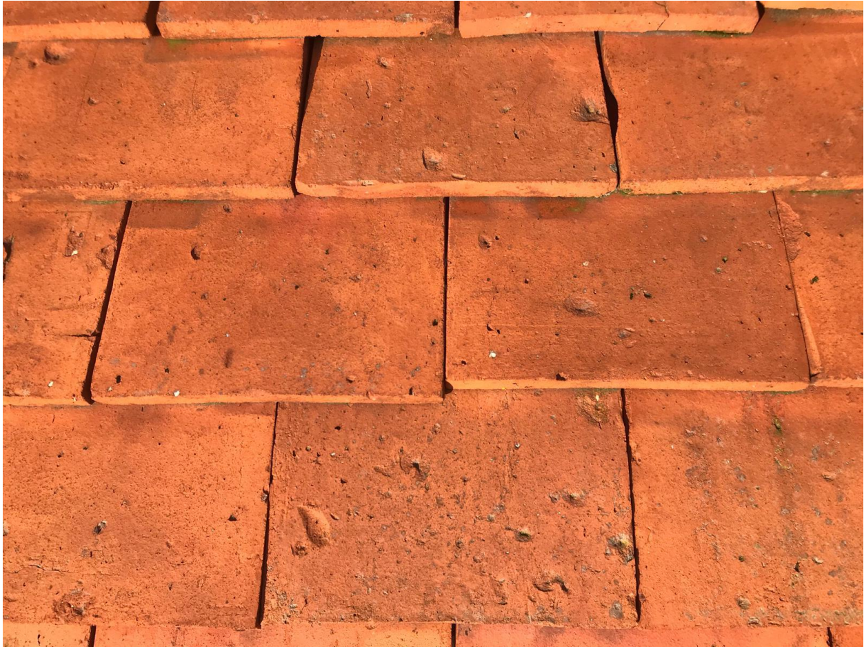
Clay tiles for roof to match existing barn
