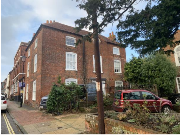
Figure 5: View of dwelling from Queen Street.
