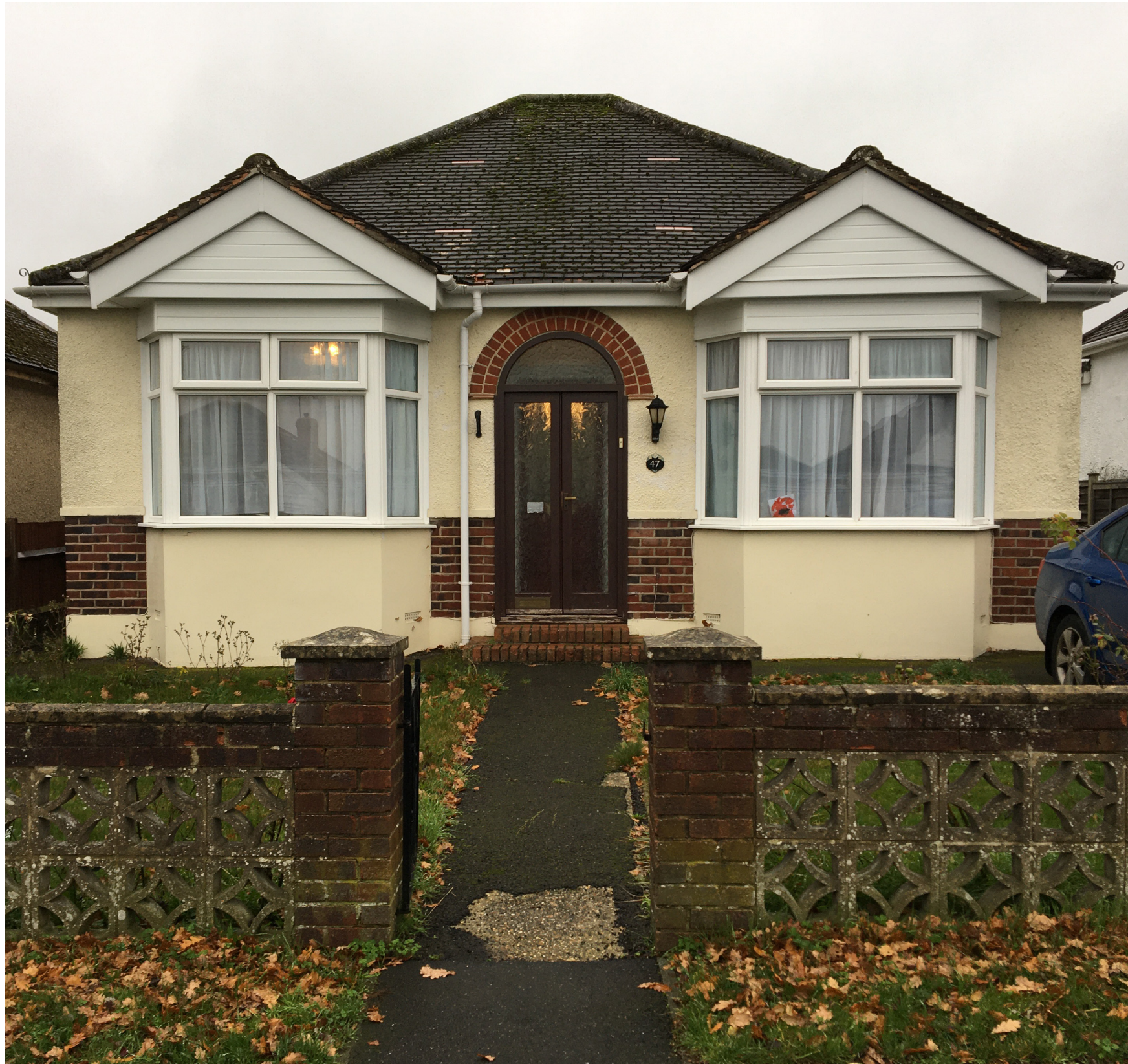
47 Maylands Road - Existing House
