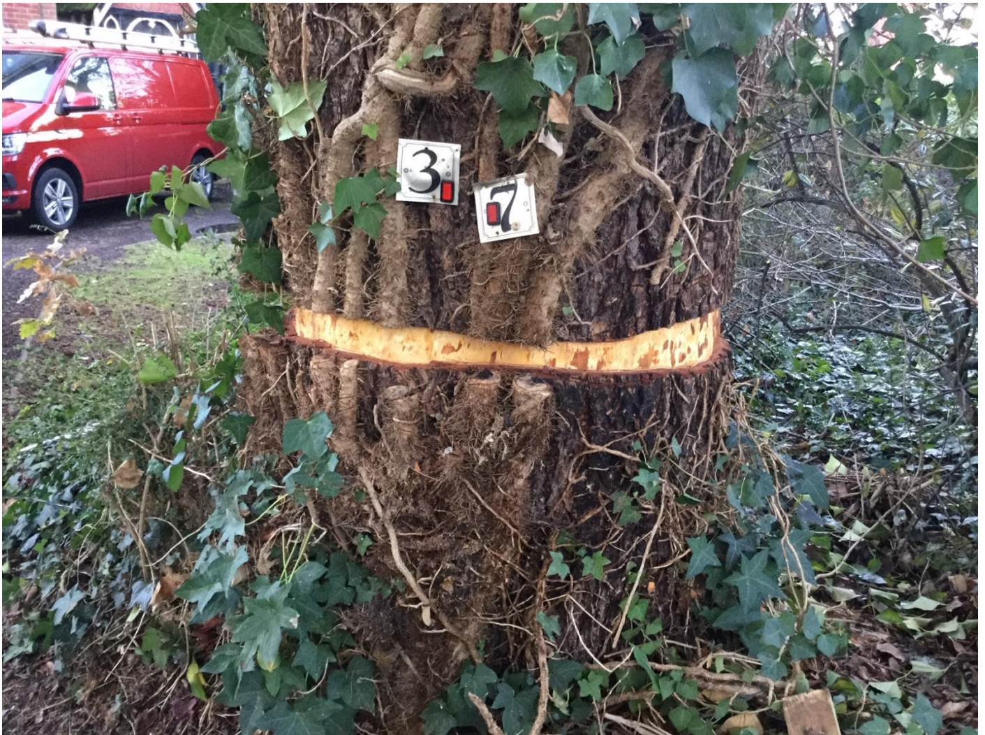
SAL2 Ivy and bark removed at c1m on T1 cedar with the cut into the sapwood being c2mm wide and c2 to 3mm depth.
