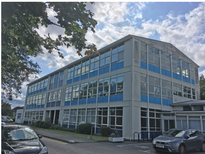
Fig 3: NE corner of 3 Storey Block
