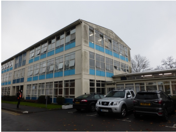
Fig 12: Elevation showing the quantity of modern top hung window replacement - 3 Storey Block
