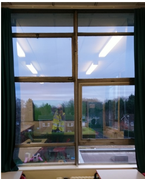
Fig 14: Internal image to show modern top hung window replacement - 3 Storey Block
