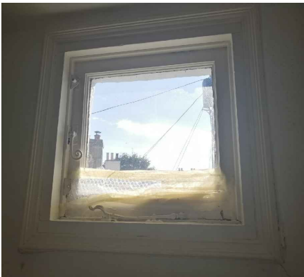
W2 - Photo of existing window
