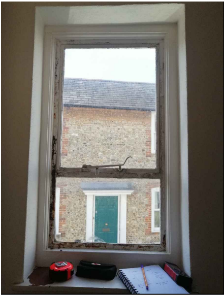
W1 - Photo of existing window
