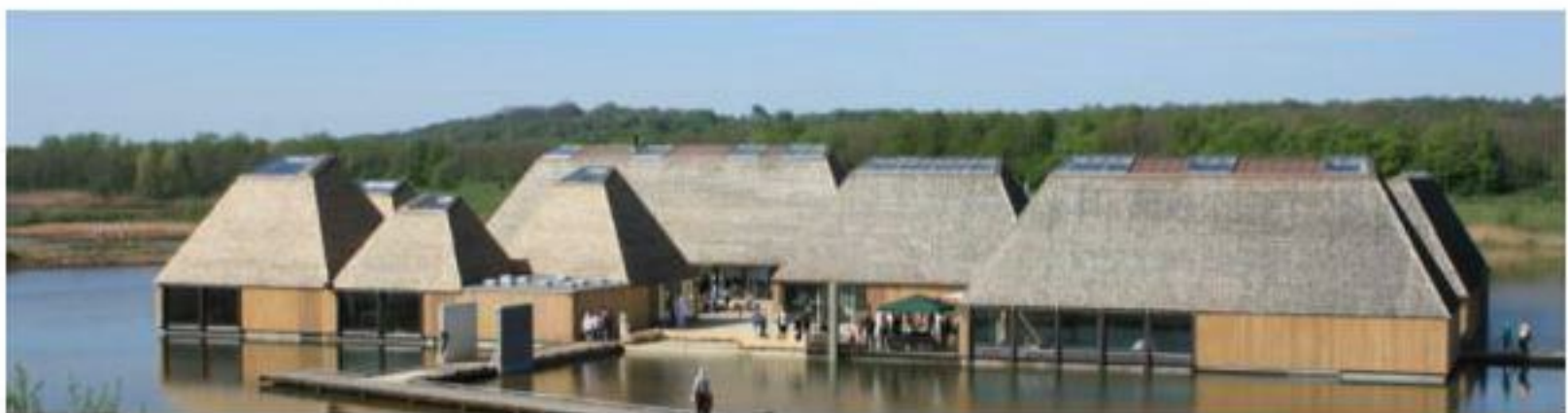
Brockholes a floating visitor centre, Lancashire Wildlife Trust
