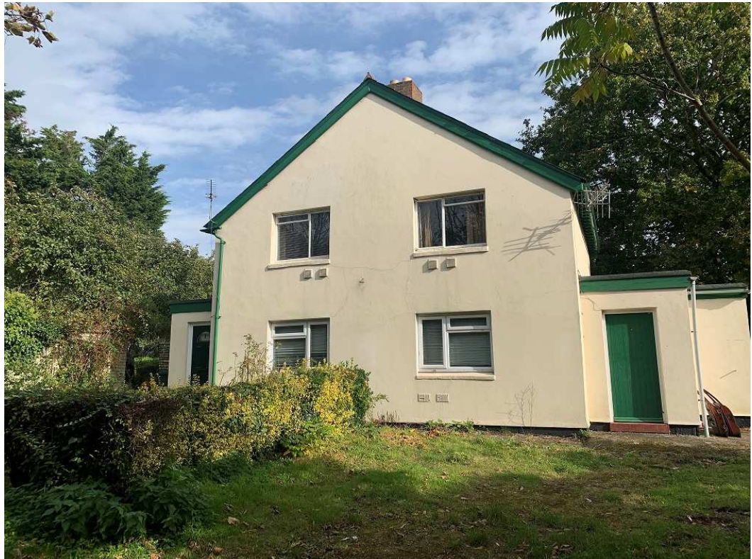
Photograph showing the existing front elevation
