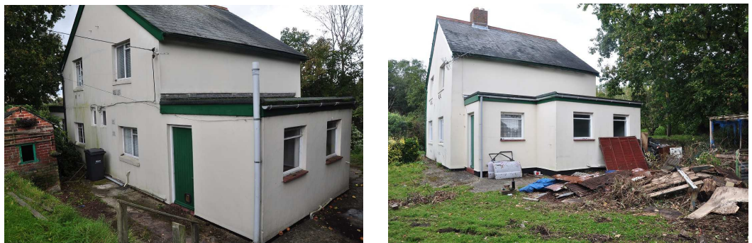
Photographs showing the existing rear and side elevations
