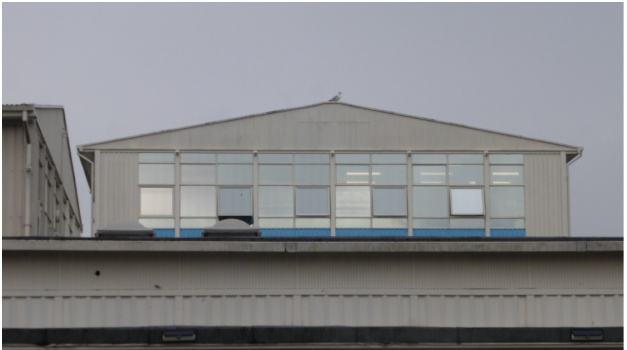
Fig 22: South elevation of 3 Storey Block (Building ref "A")
