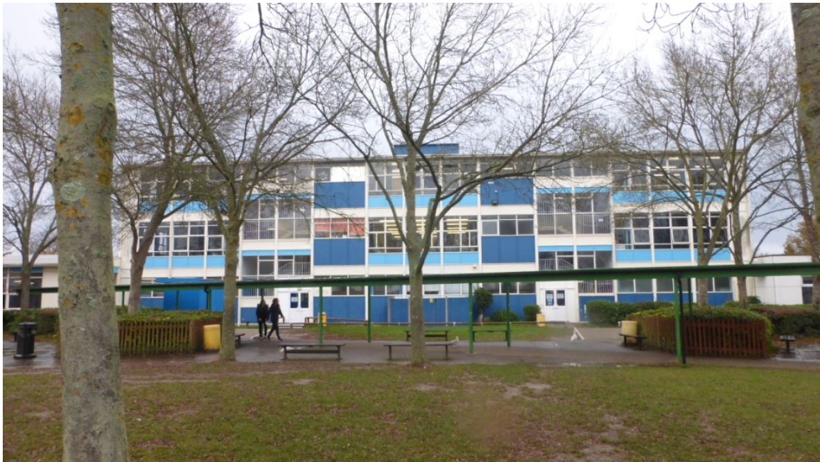
Fig 2: West Elevation of 3 Storey Block (Building ref "A")
