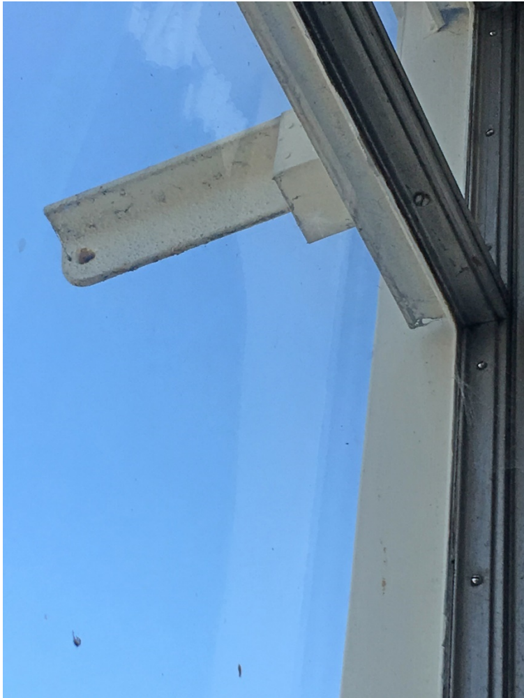
Fig 7: External eaves level bracket– 3 Storey Block
