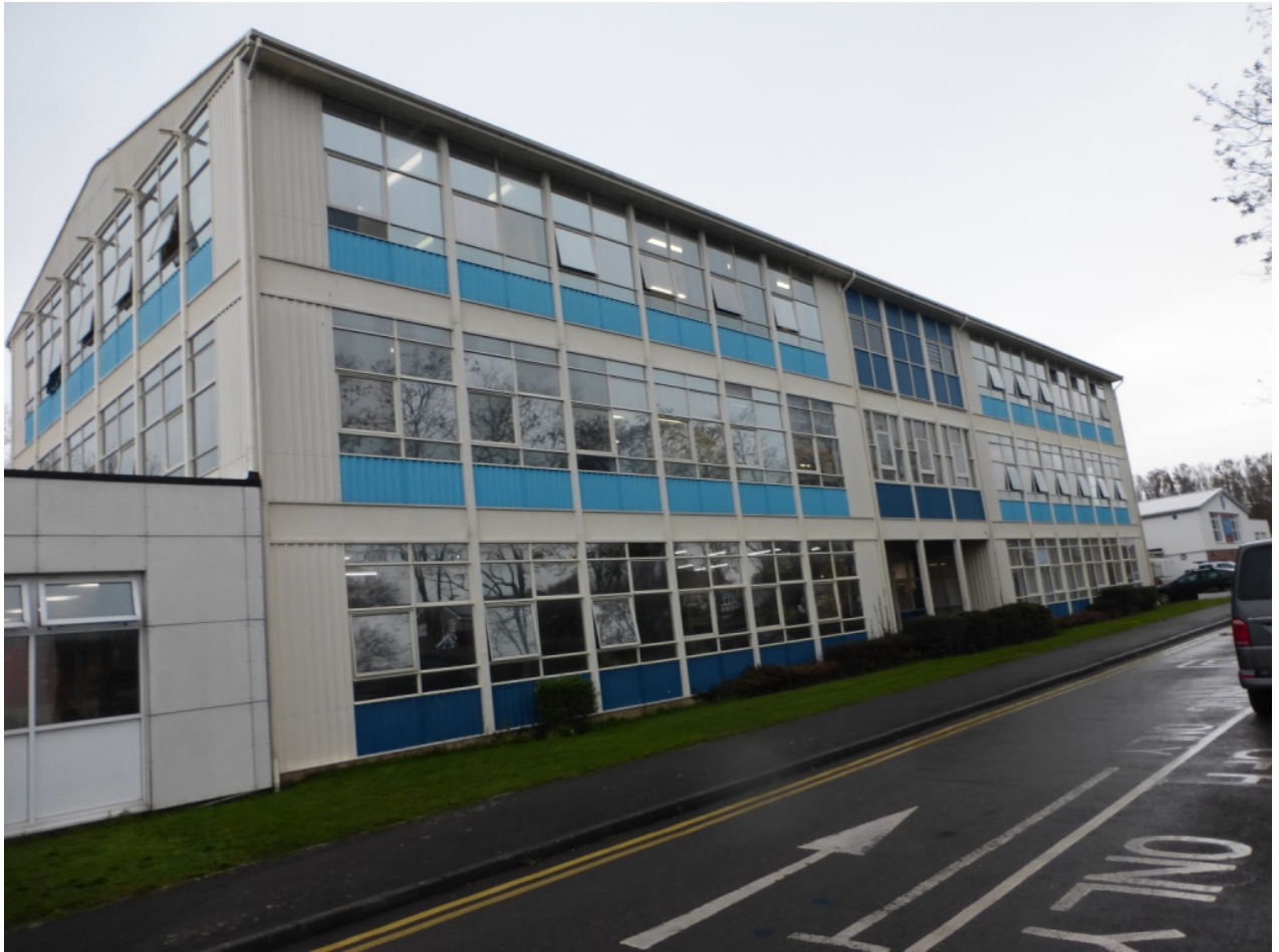
Fig 21: SE corner of 3 Storey Block (Building ref "A")
