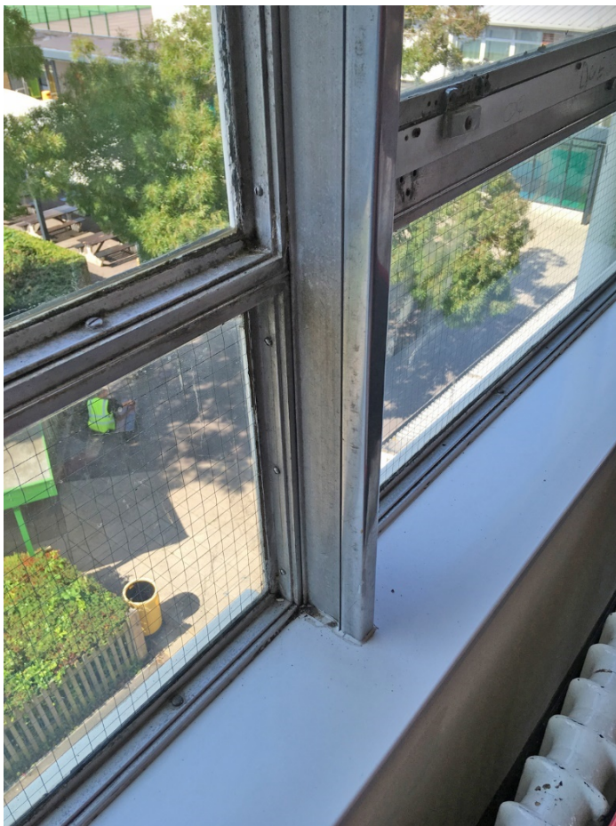
Fig 5: Aluminium Mullion / Transom / Cill detail – 3 Storey Block
