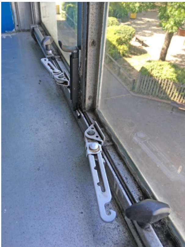
Fig 11: Original casement window, with modern window restrictors - 3 Storey Block
