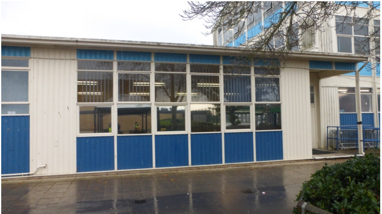
Fig 20: West Elevation - Single Storey Reception (Building ref "C")
