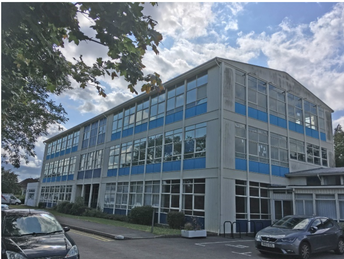
Fig 3: NE corner of 3 Storey Block (Building ref "A")
