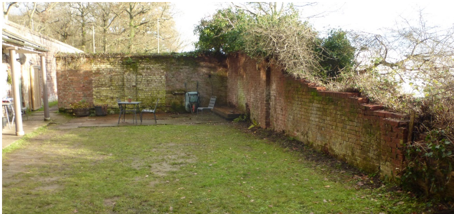
Fig 7: North wall viewed from within Stable Cottage garden
