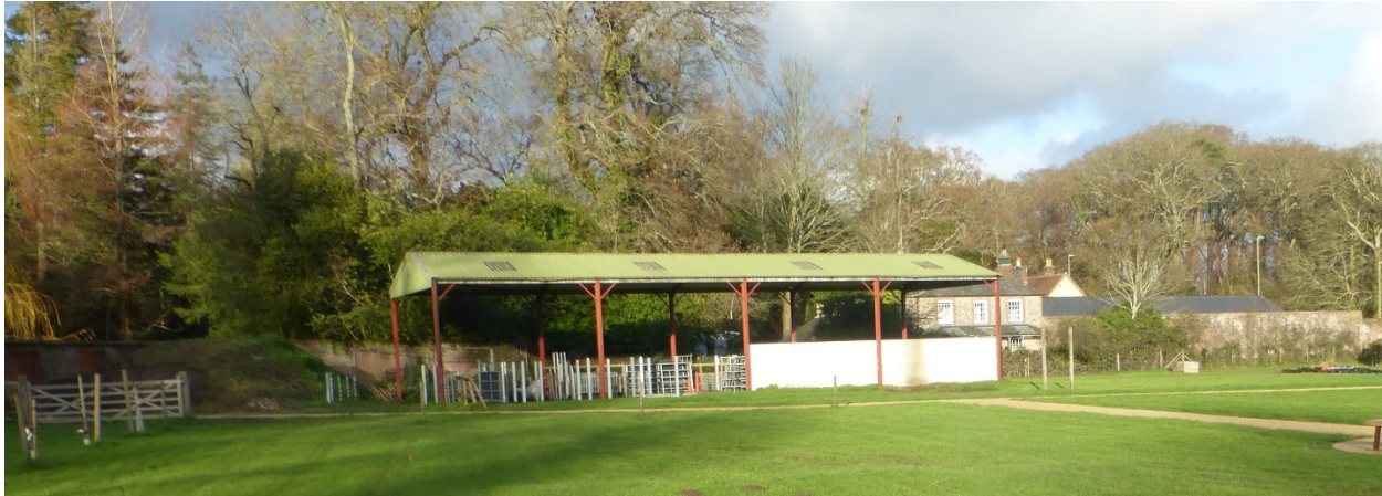
Fig 5: North wall South elevation viewed from Storey Gardens
