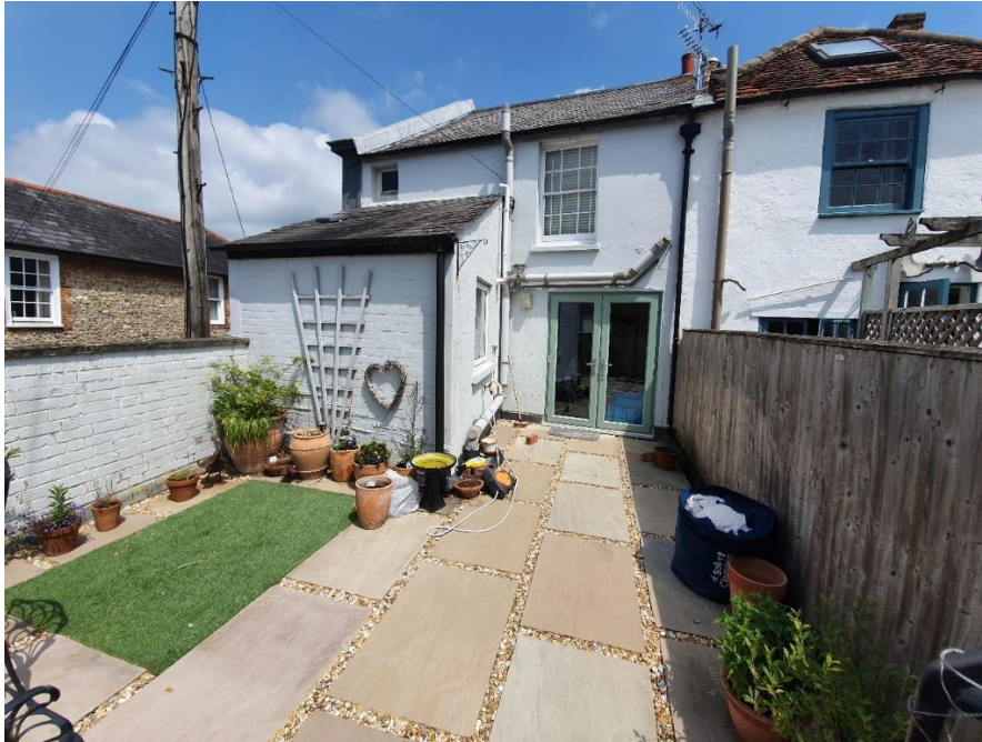
Existing first floor terrace
