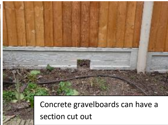
Cut a gap out of the gravel board
