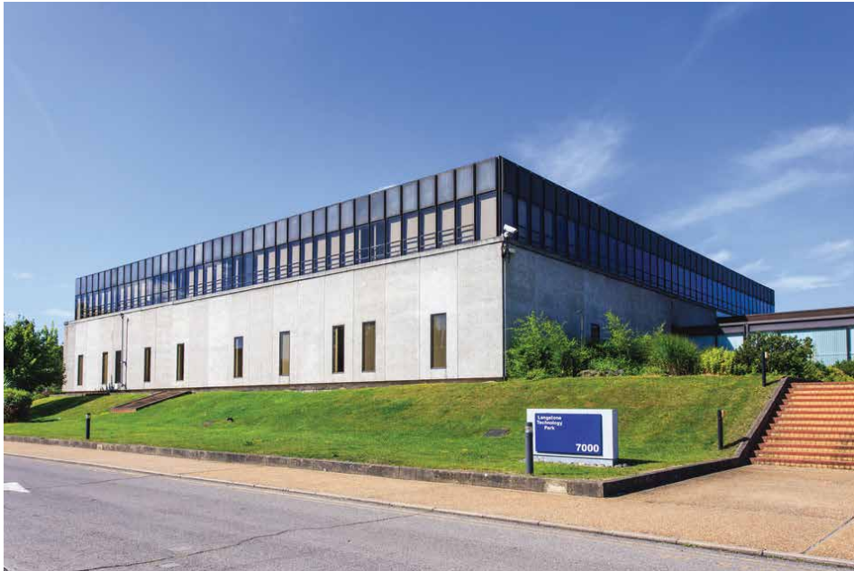
4. View from estate road toward Building 7000
