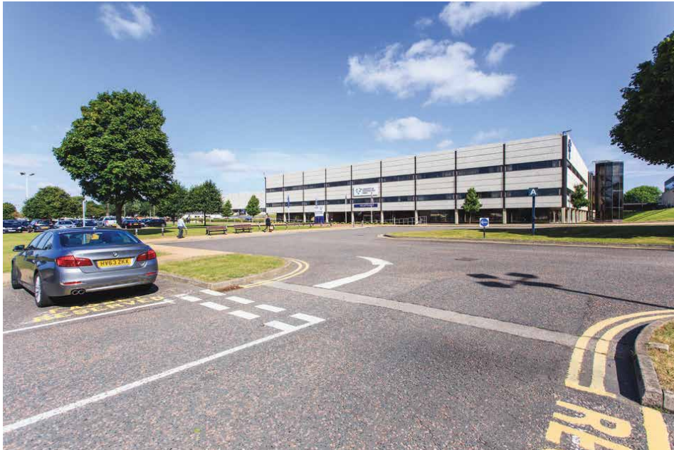
3. View from estate road toward Building 6000
