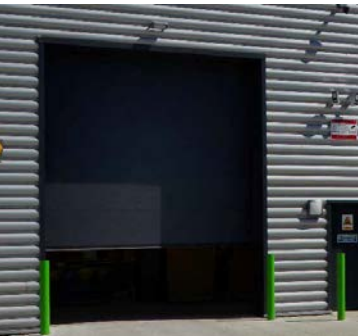
LOADING DOOR & STEEL BOLLARDS
