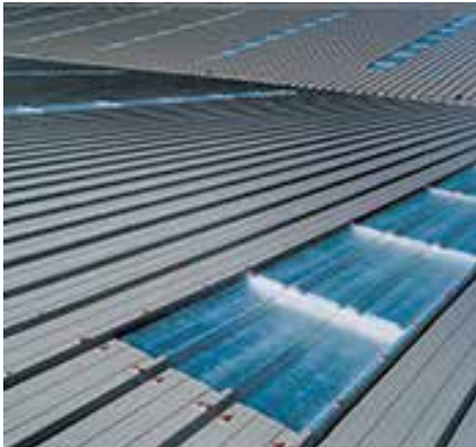
OPTIMISED ROOF LIGHT AREA
