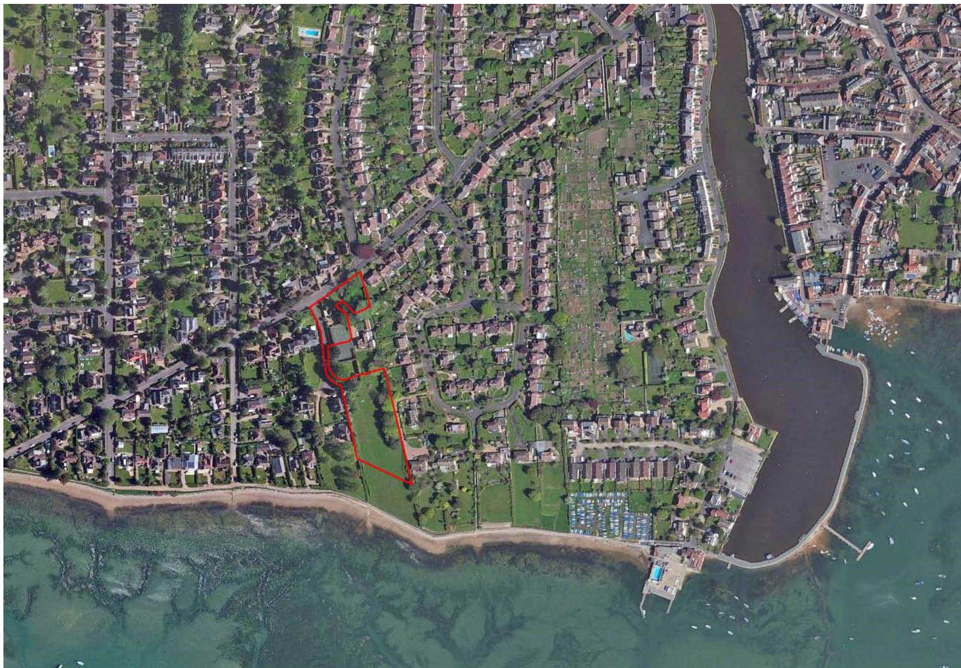
above Aerial view of site location
