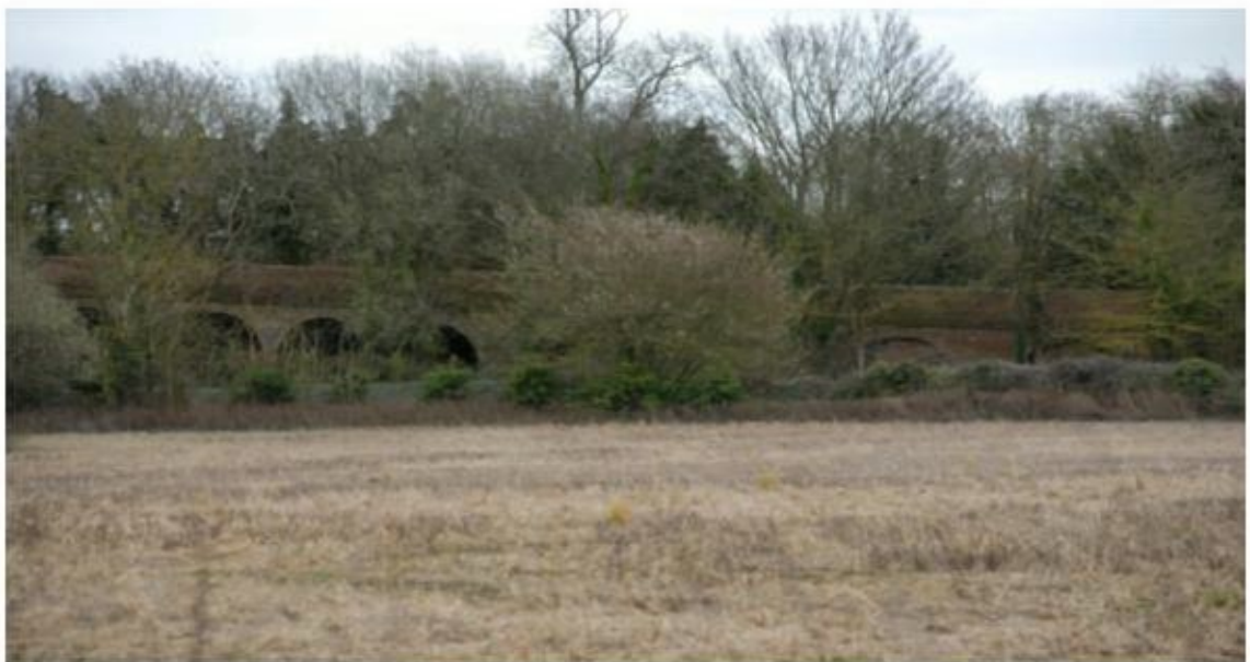
Mill Lane Bridge from Lower Road.
