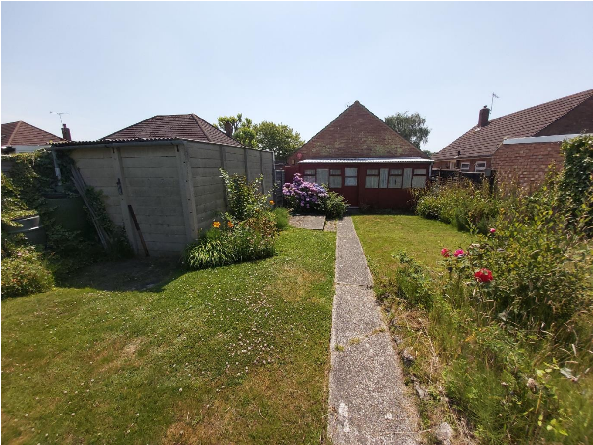
Photo 2: Rear of property
