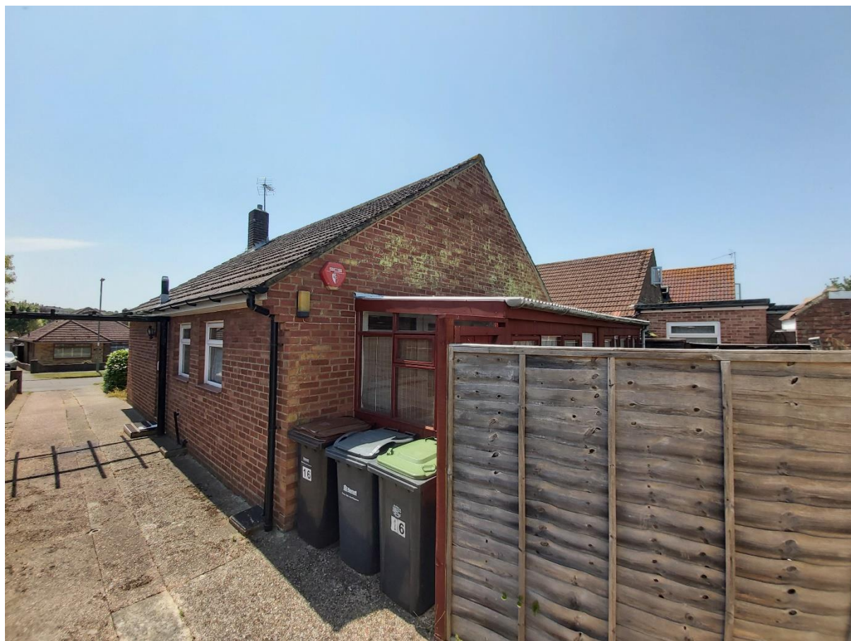
Photo 4: Rear of property
