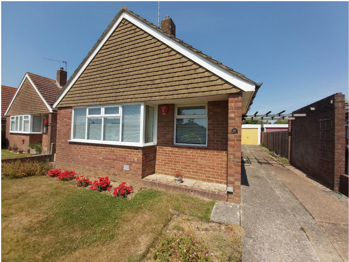
Photo 5: Front of property
