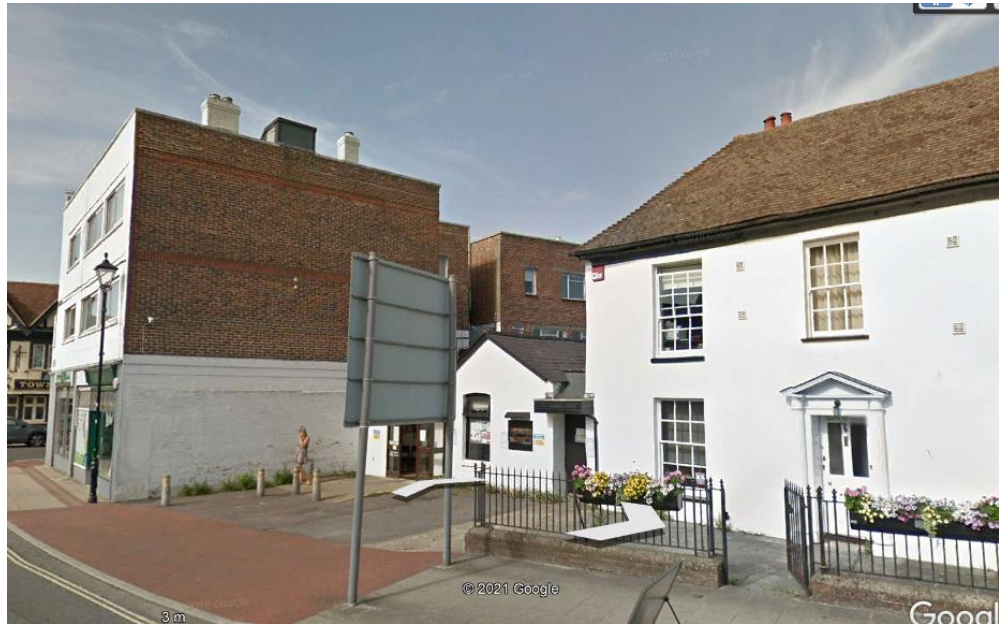
Figure 1 The three-storey wall of the Central Buildings adjacent to the site
