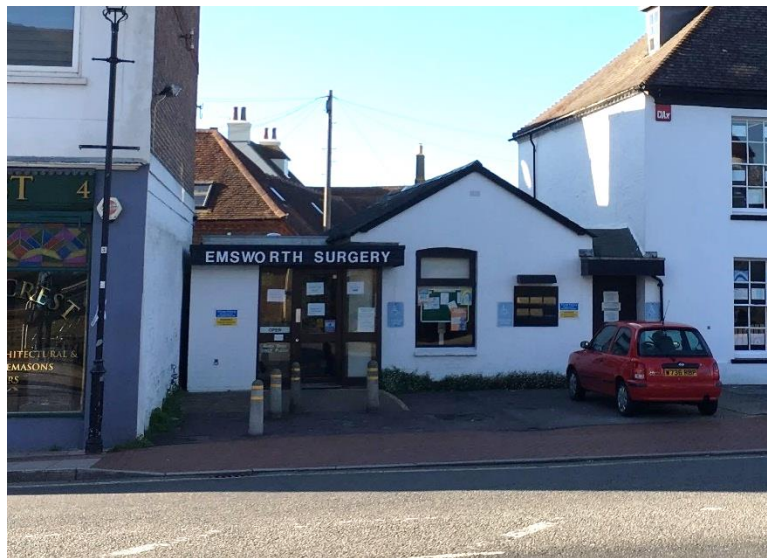
Figure 3 The southern façade of the Listed building
