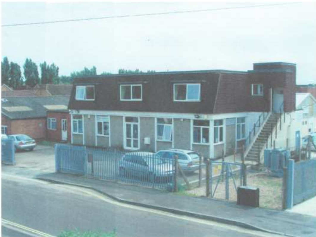
Archive photograph of Jubilee House taken from the first floor of a dwelling opposite the site. The ground floor section of this building has had a new face lift since this photo was taken.
