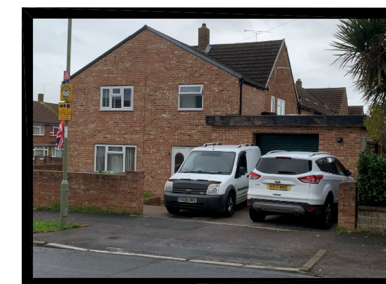
Photo - North Elevation
