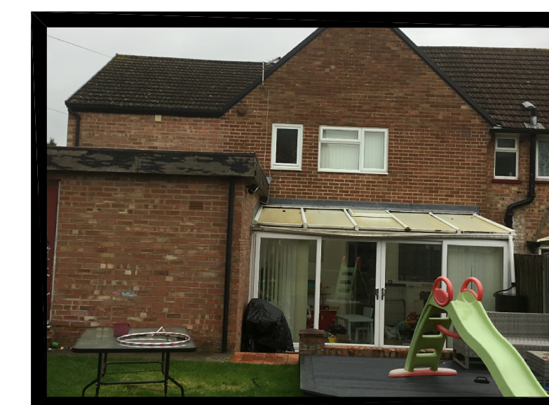
Photo - West Elevation
