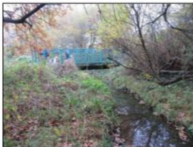
Figure 15: Riders Lane Stream where the pipeline crosses this watercourse (Section G)
