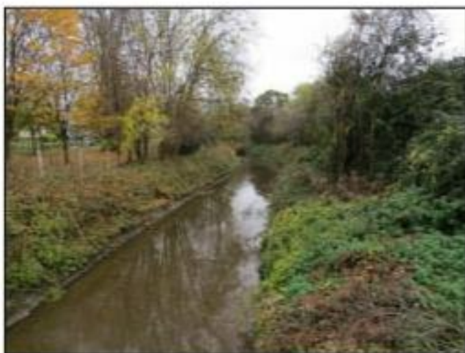
Figure 14: Hermitage Stream south of Corhampton Crescent showing concrete stream bed and banks
