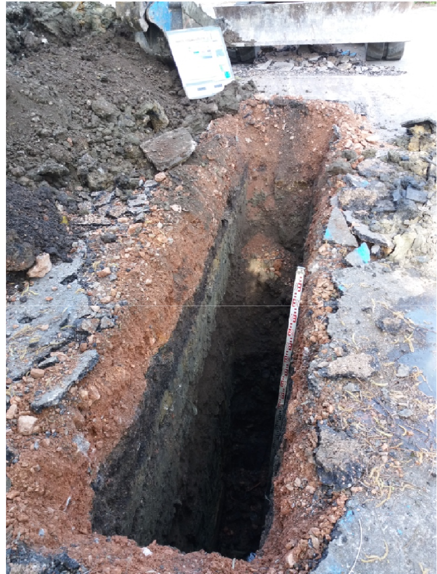
TP09 Pit – General View
