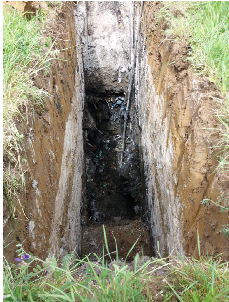
TP11 Pit – General View
