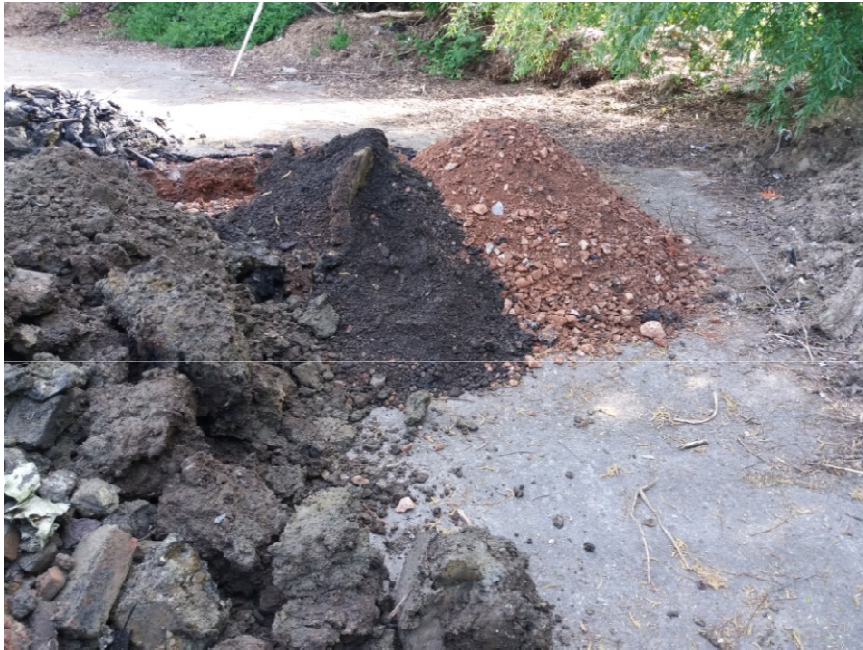
TP09 Pit Spoil – General View
