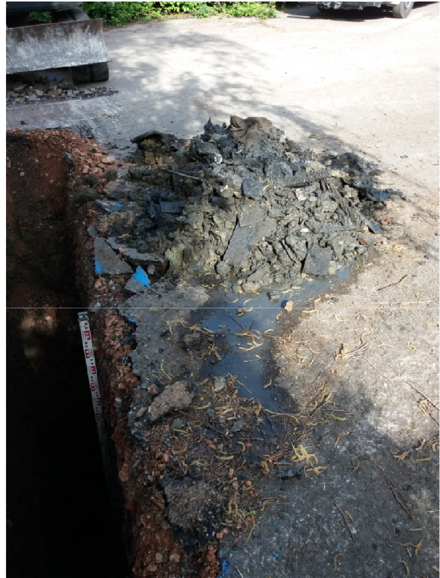
TP09 Pit Spoil – Landfill Material
