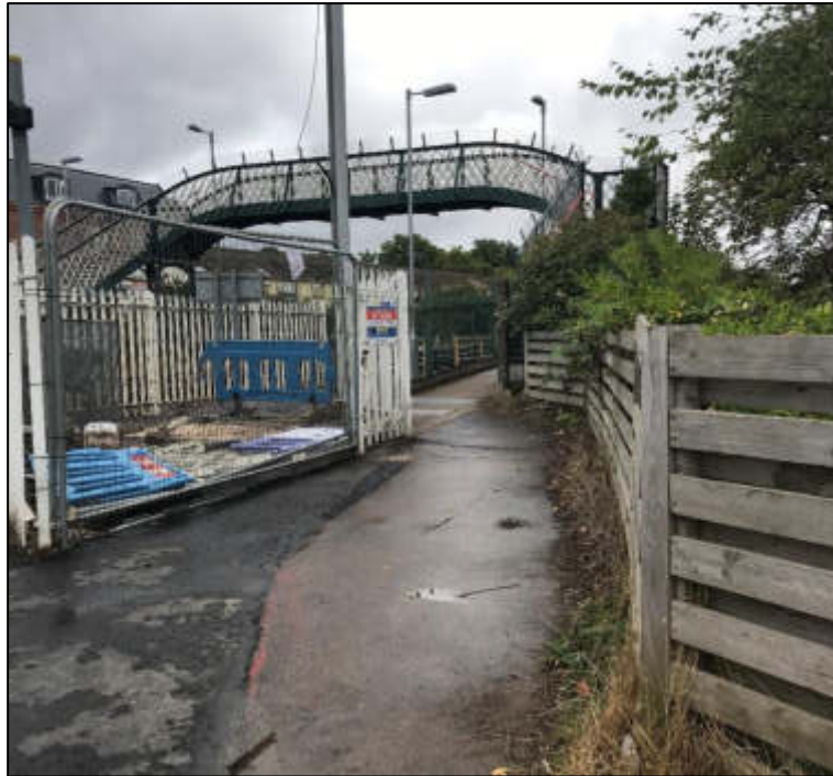
Image 1: New Lane Pedestrian Footbridge
