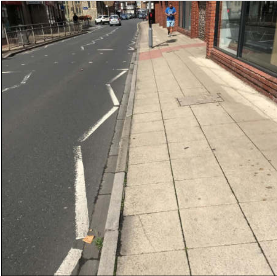
Image 12: North Street (south facing)
