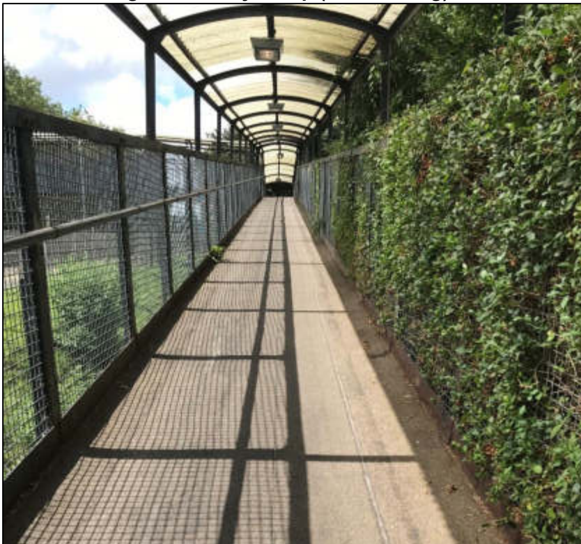
Image 9: Railway Ramp (north facing)
