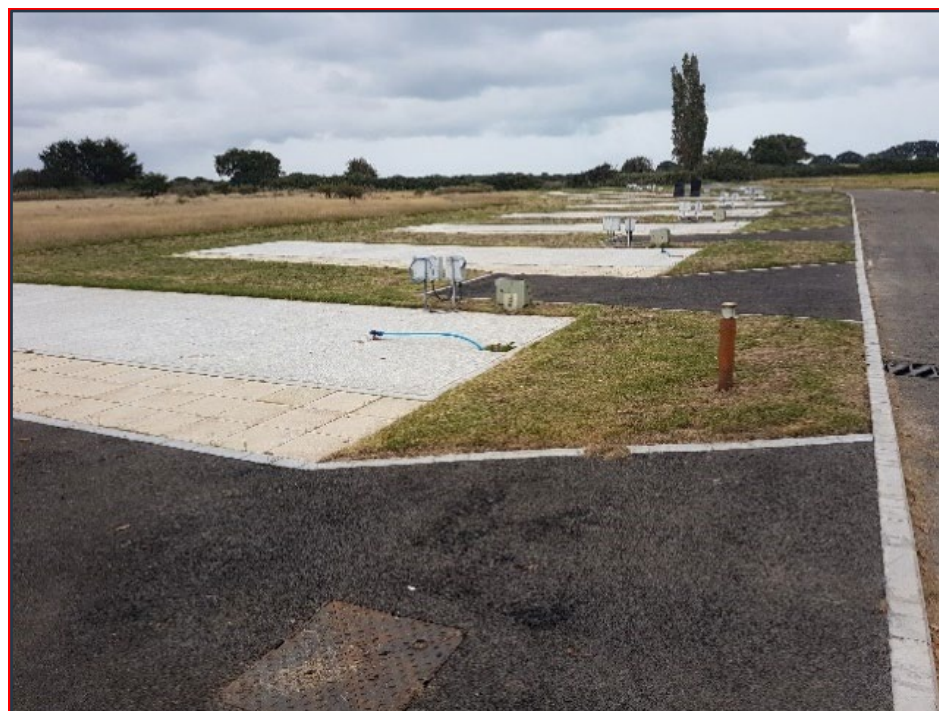
Figure 4B: Image of constructed bases
