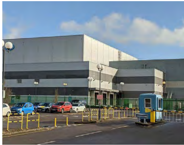
Photograph A. Structures within the Site
