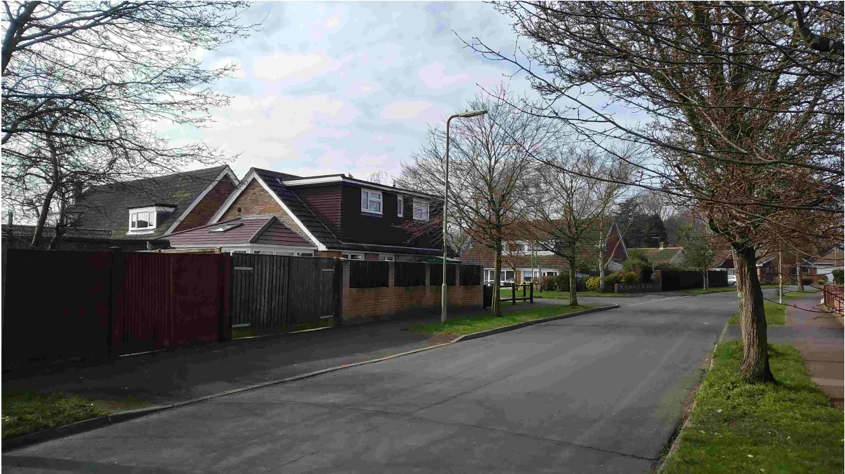
Location 9 – Full width side dormer visible from street in Sutton Road
