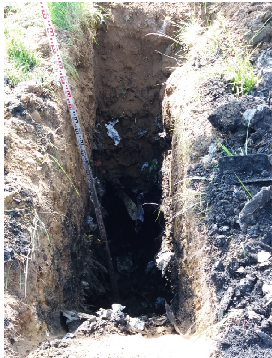
TP08 Close up of Pit Wall
