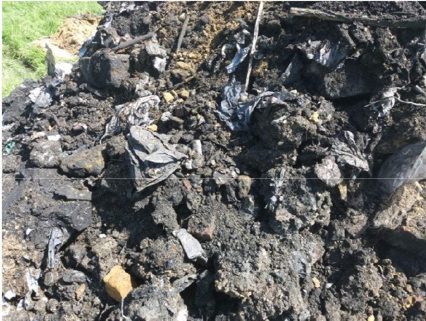
TP06 Pit Spoil – Close up of Landfill Material
