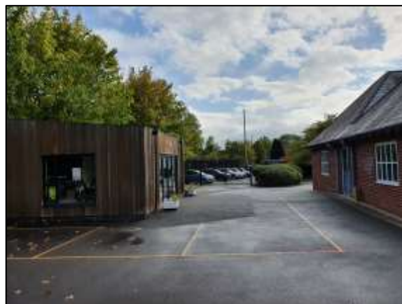
Photo 2 Hardstanding and buildings adjacent to the works footprint
