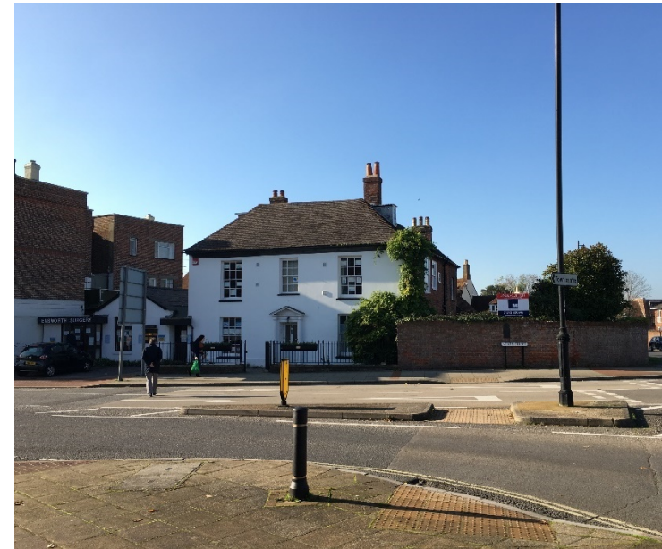
Plate 6: 6 North Street, principal east elevation.
