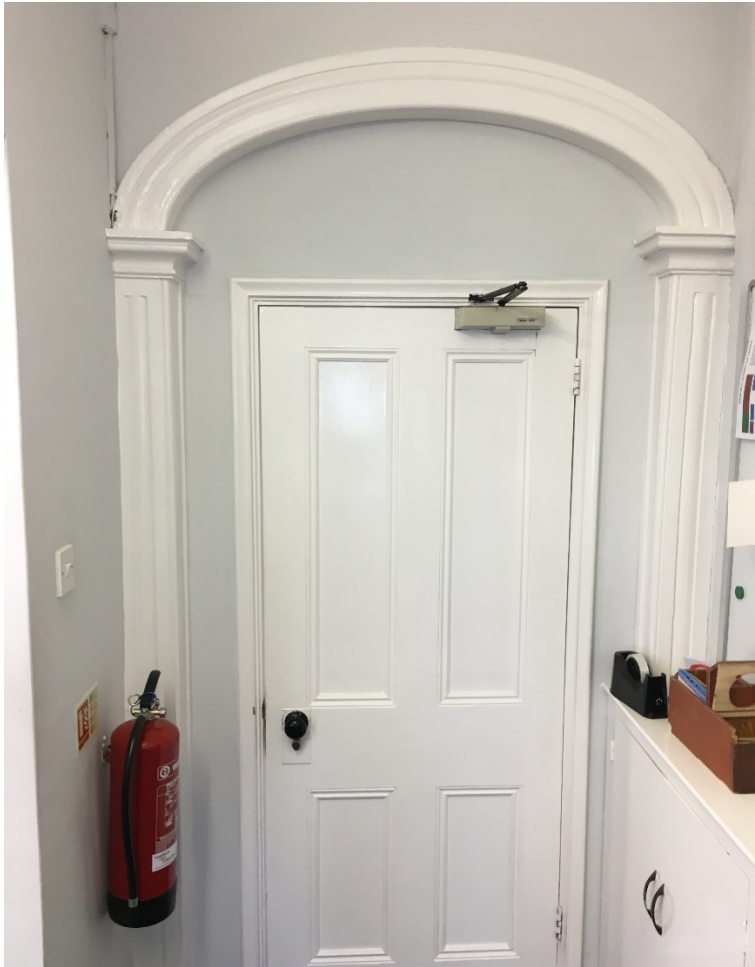
Plate 27: Architrave detailing in Room 1 (former entrance hall).
