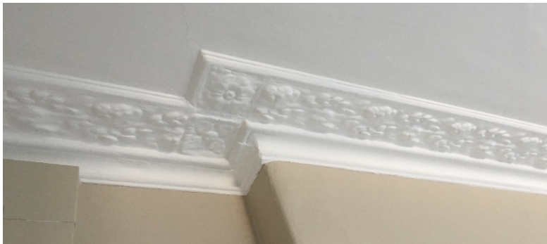
Plate 29: Decorative cornice, Room 3a.
