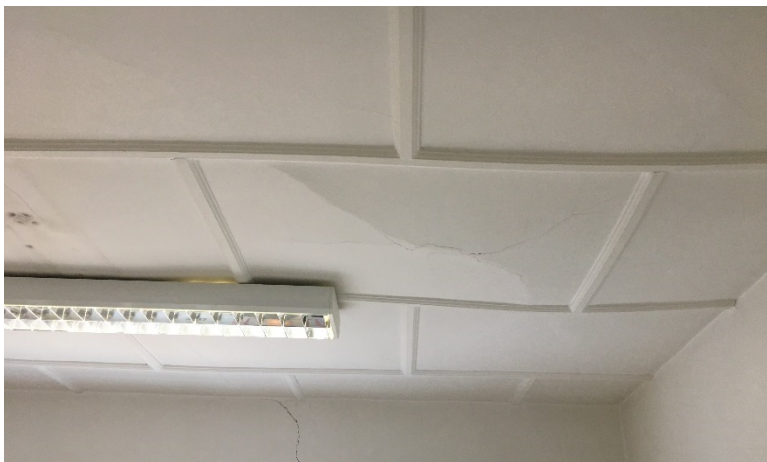
Plate 30: Panelled plaster ceiling, Room 12.
