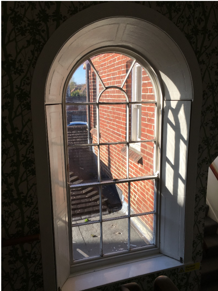
Plate 32: Window above the main staircase (Room 10).
