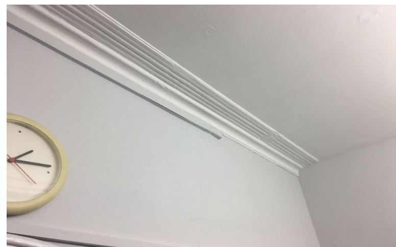
Plate 35: Moulded cornice above the partition wall between Rooms 1 and 3b.
