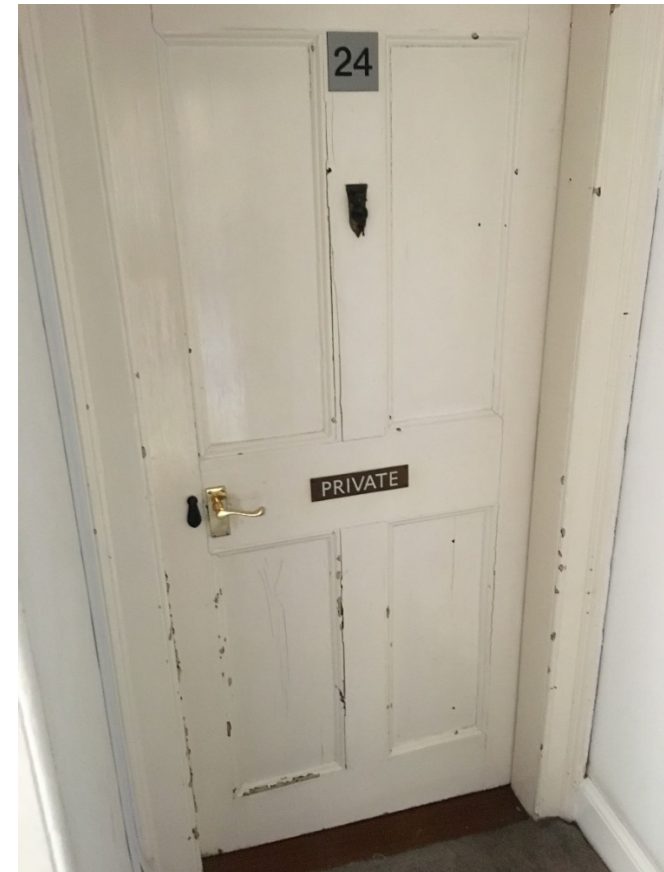
Plate 31: Door to Room 15 (labelled 24) from Room 11.
