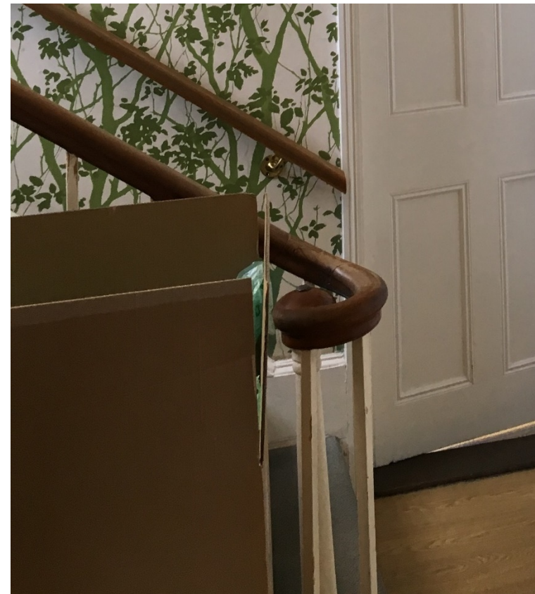
Plate 24: Detail of staircase handrail.
