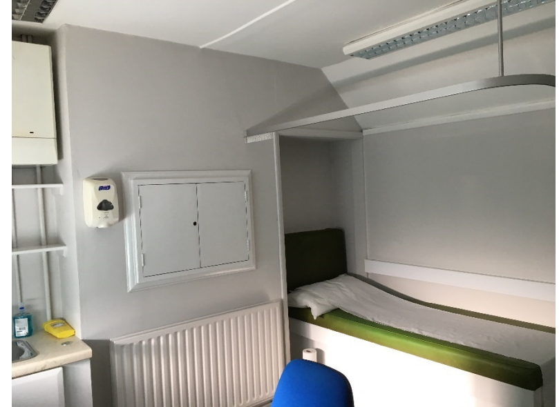
Plate 38: General view of Room 9.
