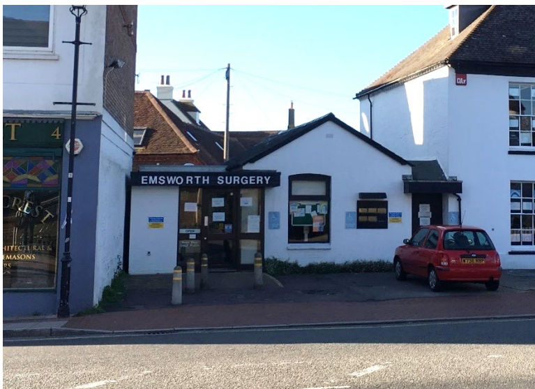
Plate 15: Detail of single-storey extension to the principal east façade.
