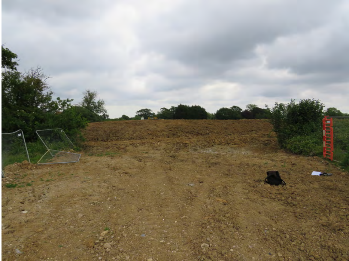
Photo 6: Looking east at break created across bramble-lined ditch to create temporary haul road (target note 17)
