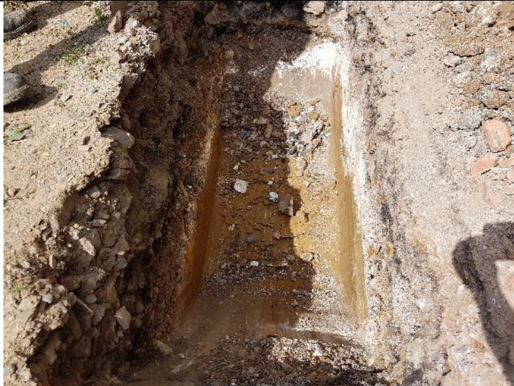
Plate 5 – TP03 – Trial pit
