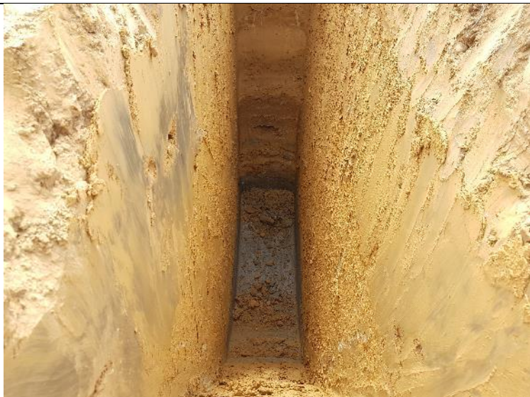
Plate 1 – TP01 – Trial pit
