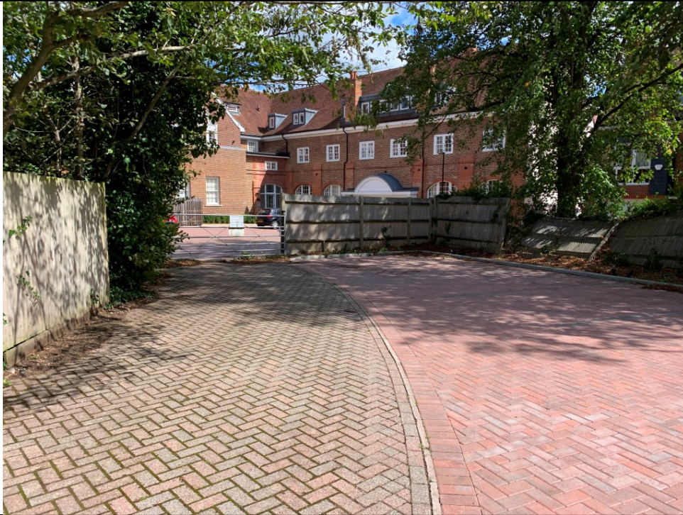
3. Car park near-complete, brick paviours used to match material and style of existing adjacent
