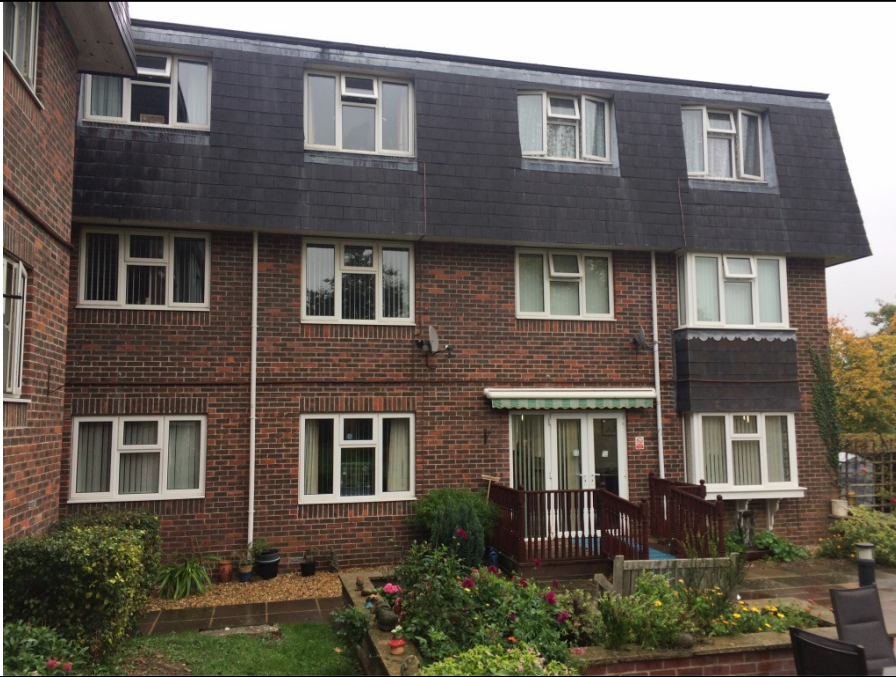
11. Rear courtyard and existing view of lounge doorset and landing.
