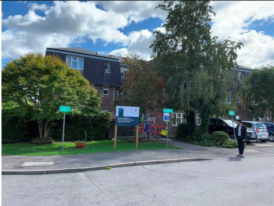
7. Front elevation of The Beeches, 1 Villa Gardens, Waterloooville. Well concealed by trees.
