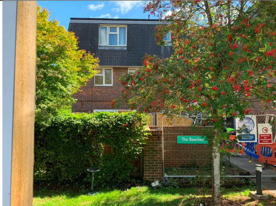
8. Front entrance approach hoarded off during works. Well screened by wall, trees and hedge.
