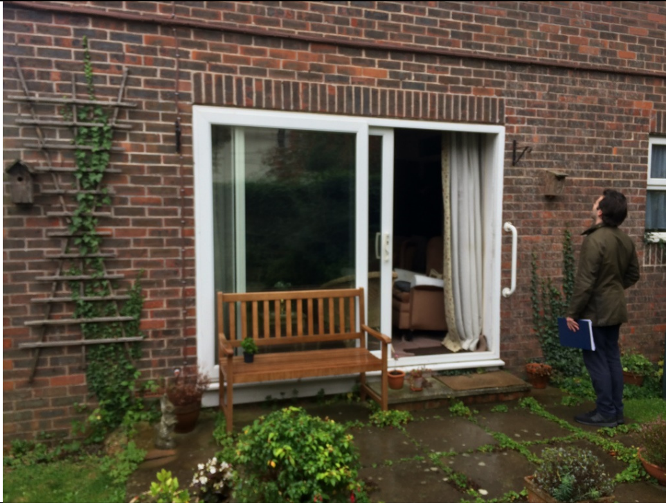
13. Front yard adjacent to front elevation and entrance pathway.
