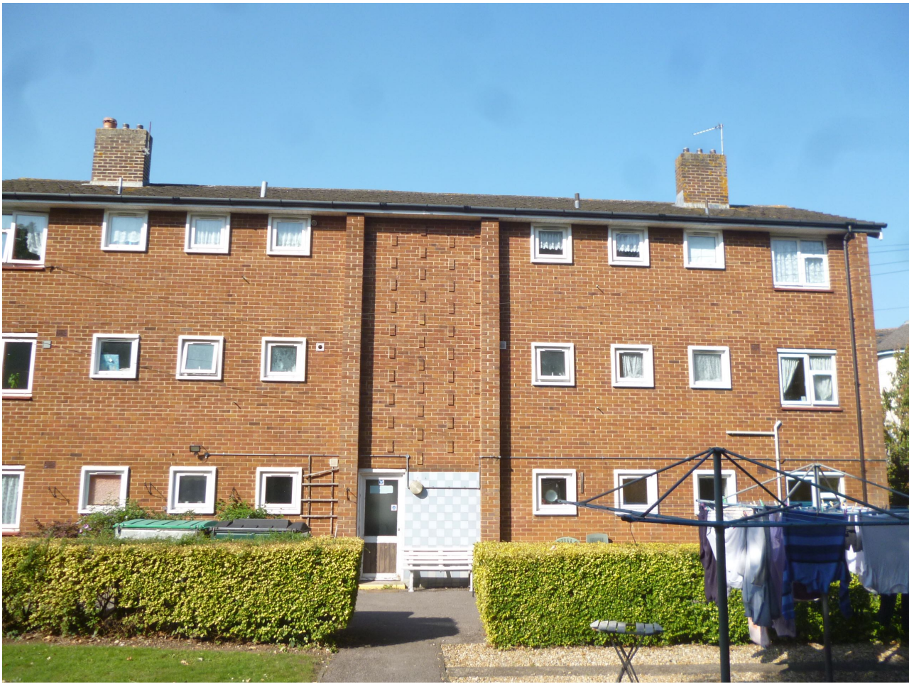
Existing Rear Elevation Image
