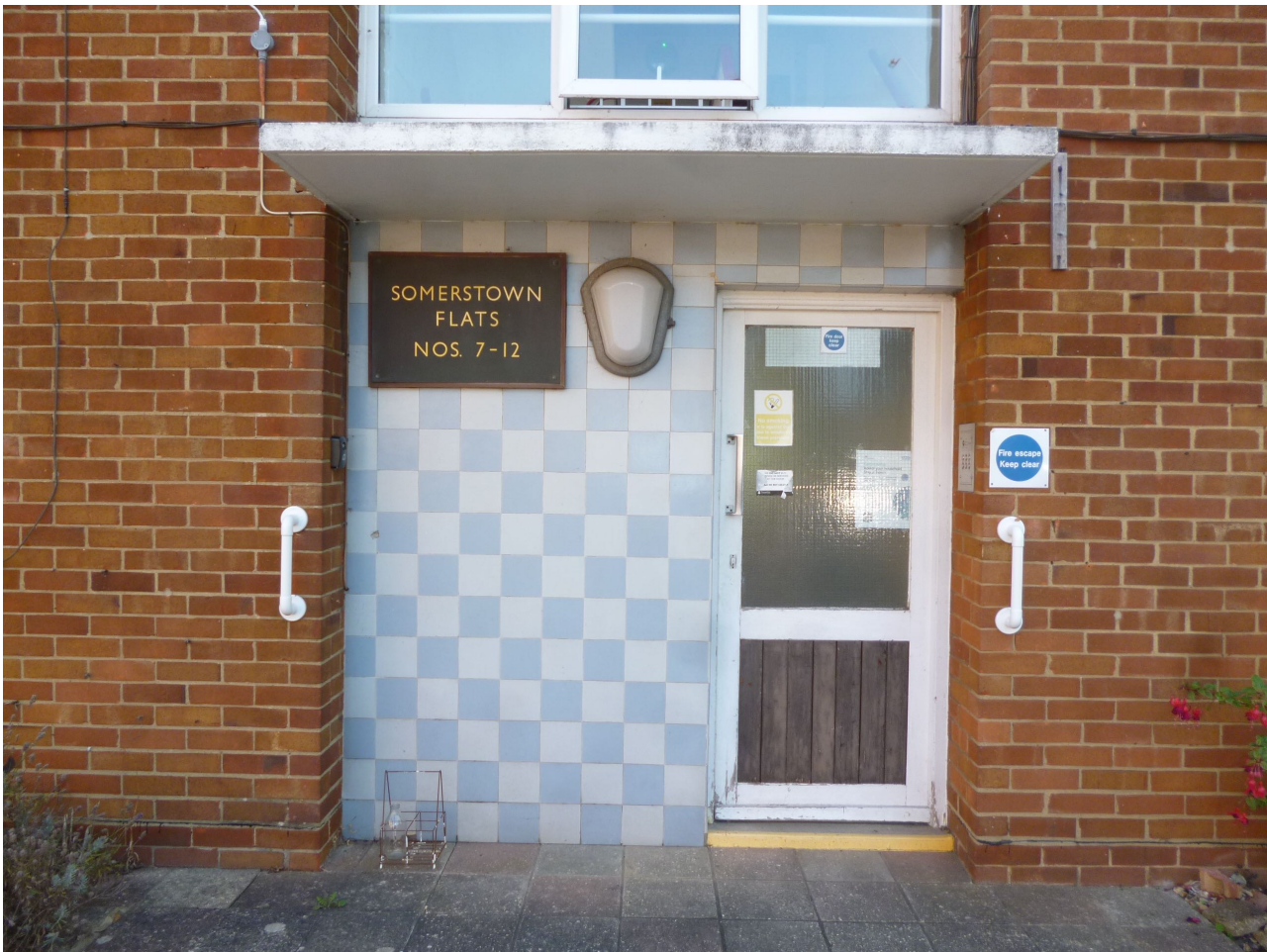
Existing Front Door Image
