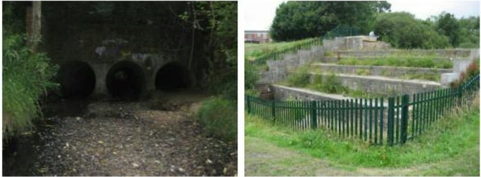
Photo 4: Major culvert & weir on Park Lane Stream
