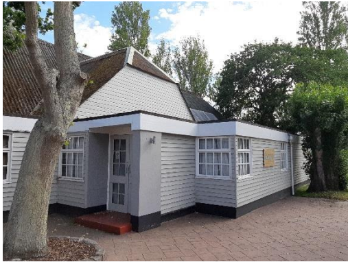
Plate 4.13: The Boathouse – north-western elevation
