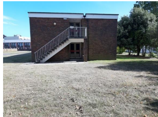
Plate 4.8: Gable end of two-storey accommodation block with access stairs
