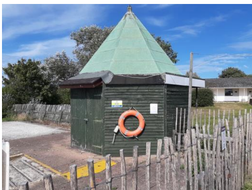
Plate 4.14: Boat House – viewed from south
