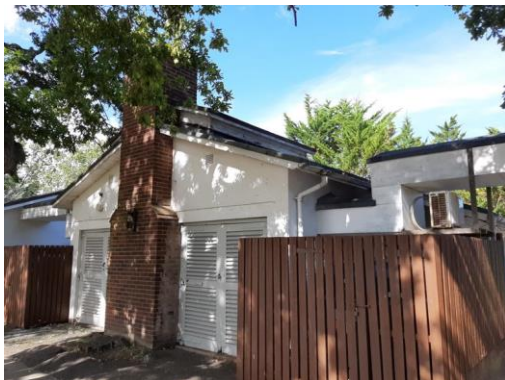
Plate 4.20: Western boiler house
