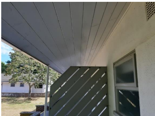
Plate 4.3: Canopy feature on frontage of accommodation chalets
