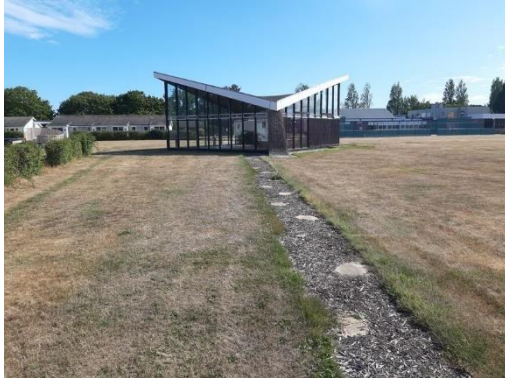
Plate 4.16: Coffee Lounge Building
