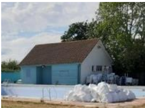
Plate 4.15: Outdoor swimming pool building
