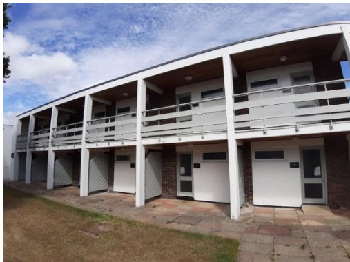
Plate 4.7: Two-storey accommodation chalets – front elevations and balcony areas
