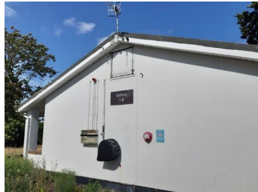
Plate 4.2: Gable end elevation with inspection hatch present in apex
