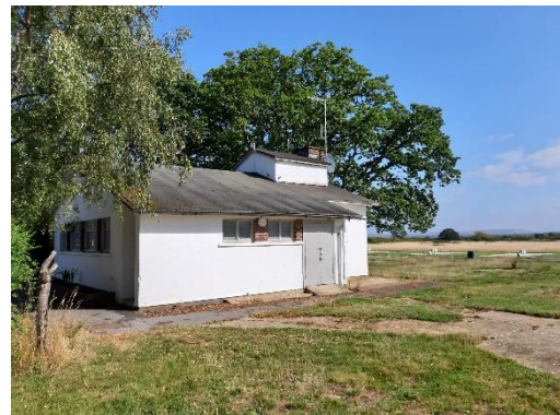
Plate 4.21: Eastern boiler house
