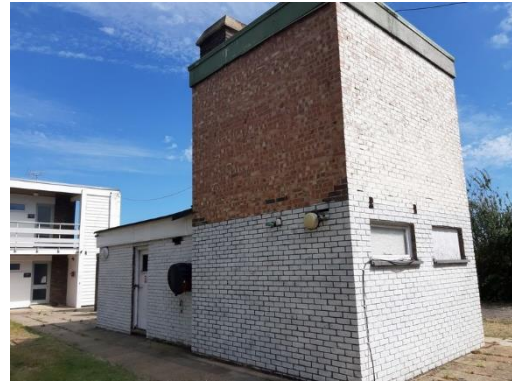
Plate 4.19: Southern boiler house – northern and western elevations
