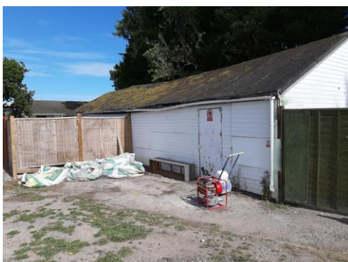
Plate 4.22: Maintenance workshop building
