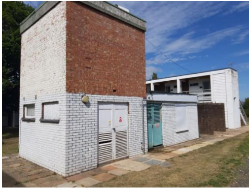
Plate 4.18: Southern boiler house – southern elevation
